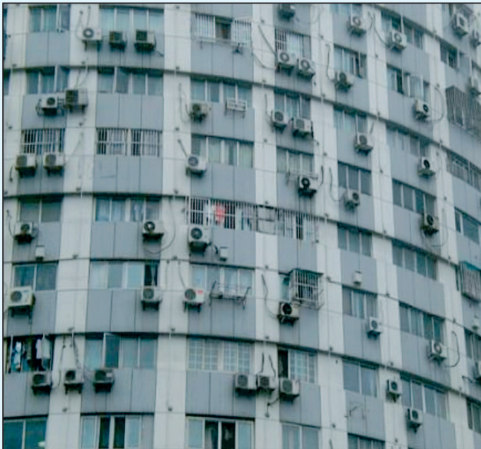
Figure 1. Split systems are façade air-conditioning systems with a condenser each mounted externally to the room for which they are active. Reference: Split System, 2014.
