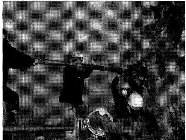
Fig 4 Installation of a reinforcing pipe containing fibres as strain sensor in the Ulsan-Kangdong tunnel.
