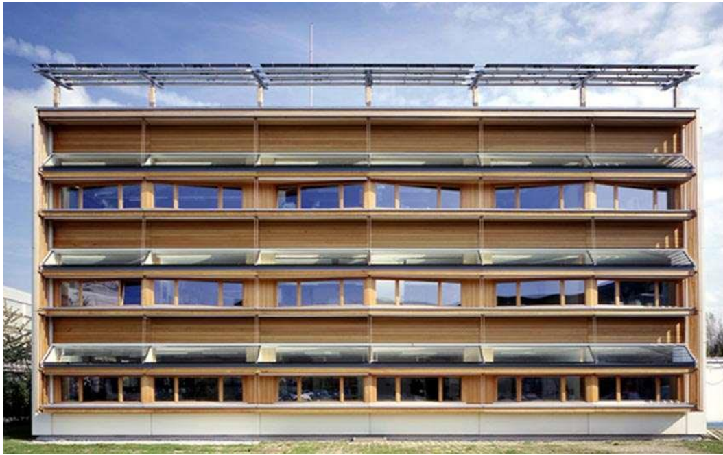
Fig. 4 - Picture of the LE South façade (credits: CHABOD Louis, 21.10.2012)
