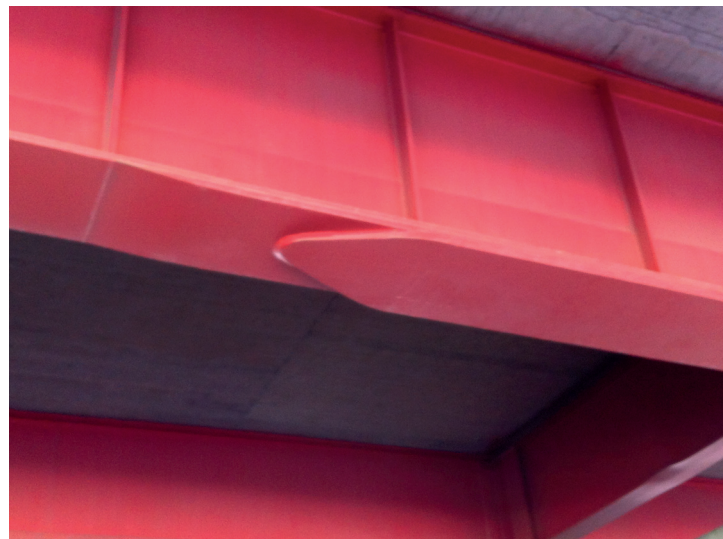
Figure 4.4: The critical detail: welded cover plate
