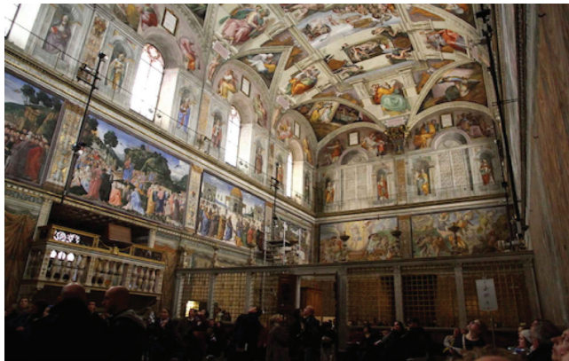
Figure 8.2 Faraday cage and network jammers installed in the Sistine Chapel to protect secrecy of the Papal conclave. Vatican, March 2013. Photo by Clayton Tang/Wikimedia Commons
