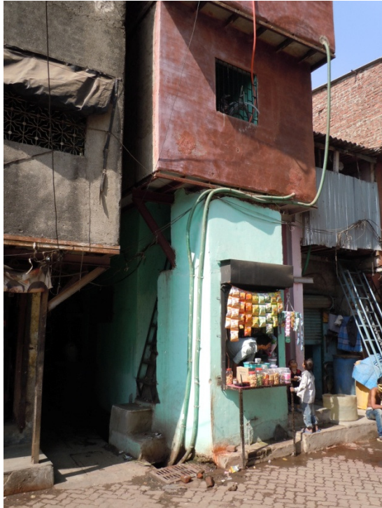
Photo 186. Stepwise encroachment on the street. Stairs and a small shop sit in front of the initial dwelling. January 21, 2013.
