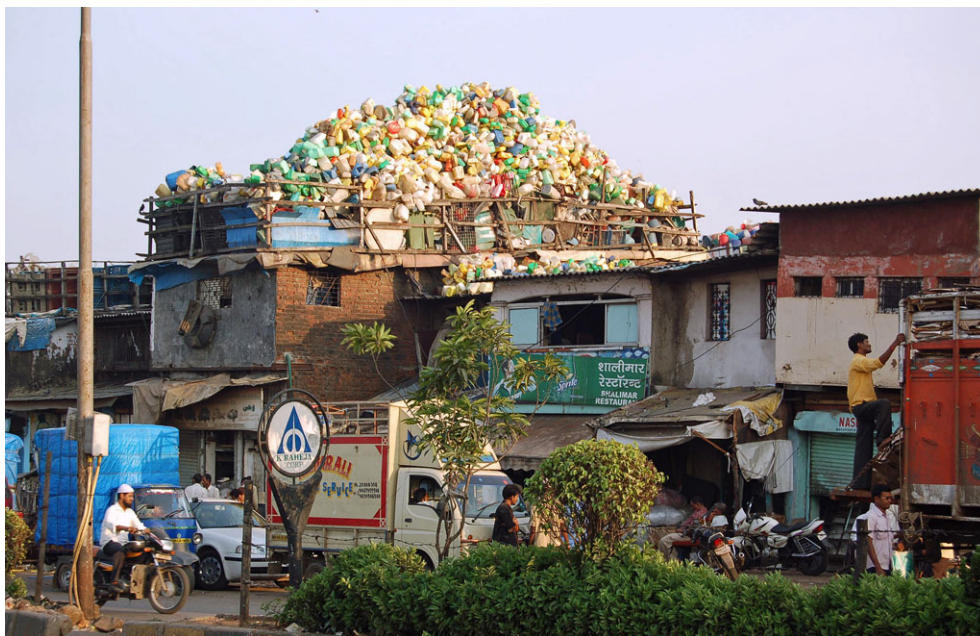
Photo 117. Plastic items are lightweight and bulky. In Dharavi's Thirteenth Compound recyclables are processed on the ground, while stock is kept on the roof. November 6, 2010.
