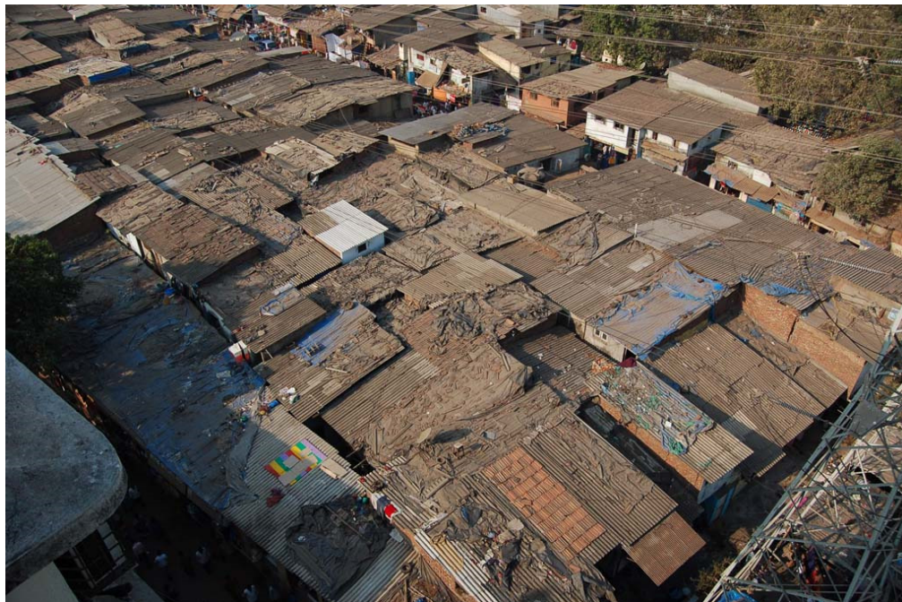
Photo 119. Asbestos-cement roofs covered with tarpaulins and roof tiles for additional waterproofing. The use of roof tiles on top of corrugated sheets, like on the house in the front, is a durable improvement of heat insulation, and slows down the spreading of asbestos fibers. Dharavi, January 26, 2010.
