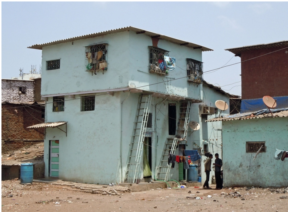
Photo 184. The overhanging upper floor gives a slum dwelling its typical mushroom shape. April 19, 2013.
