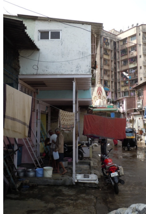
Photo 187. Encroachment on overhead space. April 10, 2013.
