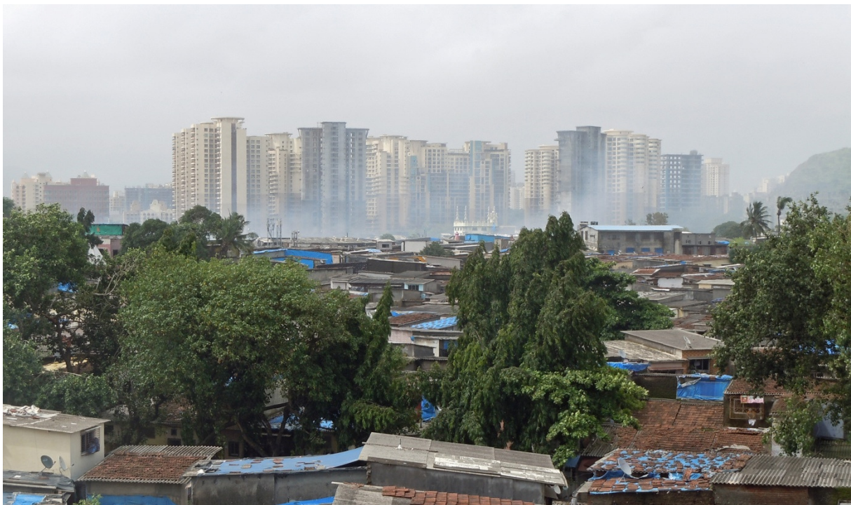
Photo 191. Slum-replacing high-rise of Nahar Amrit Shakti amidst informal settlement north of Asalpha Road, Mumbai. July 20, 2014.
