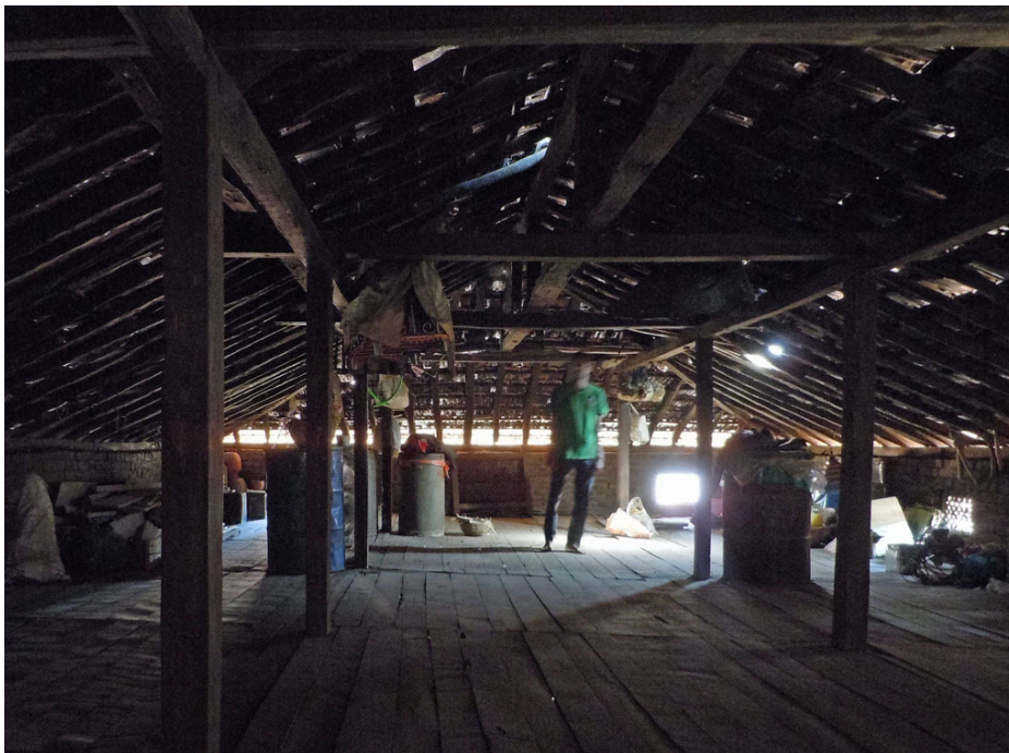
Photo 115. A tiled roof has an open structure affording natural ventilation. Interior of the house in Photo 113. November 8, 2012.
