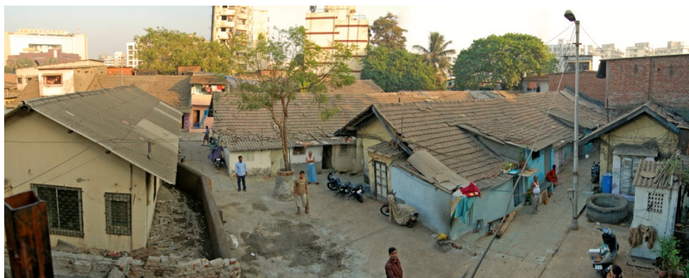
Photo 78. Chawls in Dharavi Koliwada. Verandas converted into rooms. January 13, 2009.
