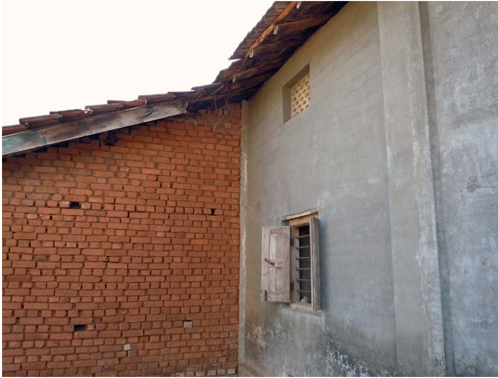
Photo 27. Kacca extension of a pucca house: earth mortar versus cement plaster. Pundhe, November 8, 2012.
