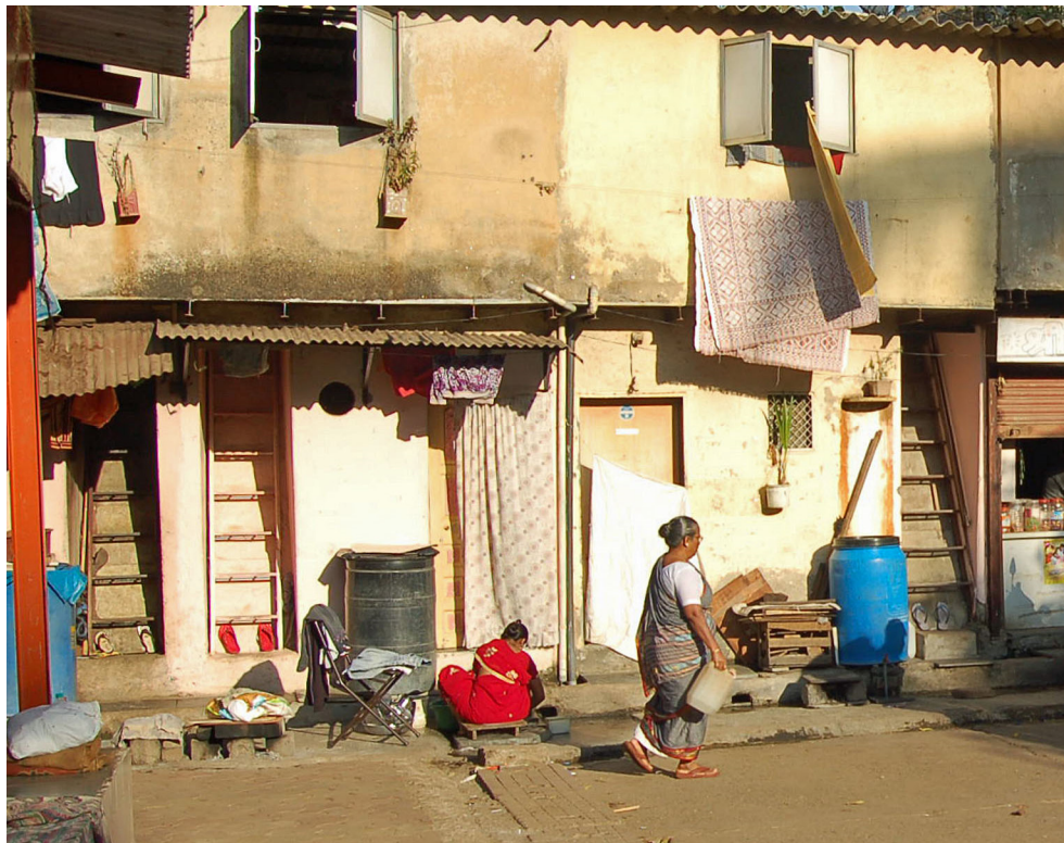
Photo 125. In Worli Koliwada, stairs sit inside the volume of the house and are part of the facade. January 10, 2013.
