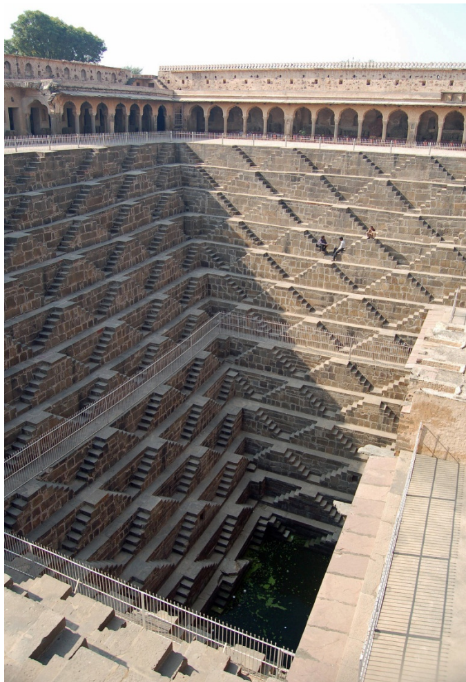
Photo 68. A step well in Abhaneri, Rajasthan, affords access to deep groundwater. Water tanks in Mumbai were less deep but played a similar important role as social hotspot. December 3, 2012.
