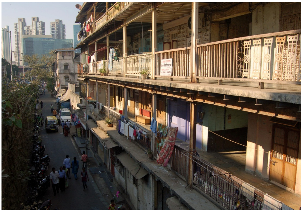
Photo 92. The single loaded corridor in a chawl is a mix of veranda and gallery. Parel Mumbai, January 6, 2013.
