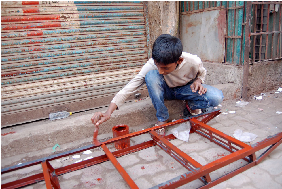
Photo 128. Stairs are of a generic design and deliverable in any color. January 17, 2013.
