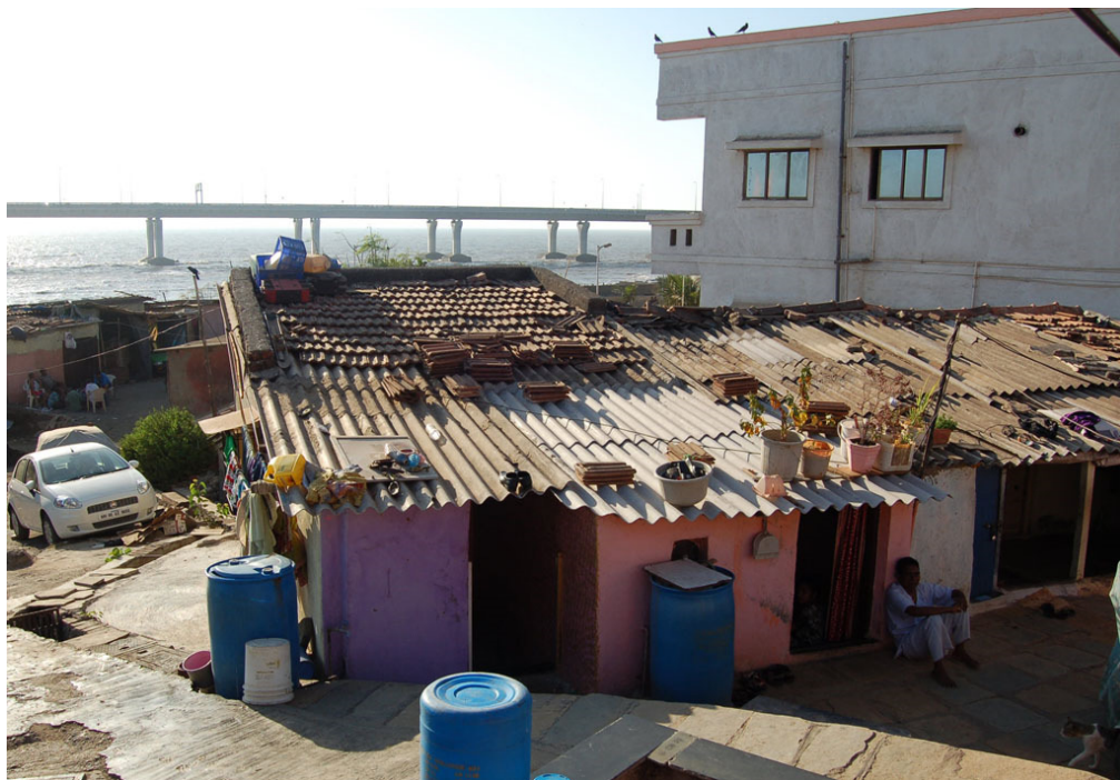
Photo 120. An asbestos-cement roof partly covered with roof tiles. Worli koliwada, April 7, 2013.
