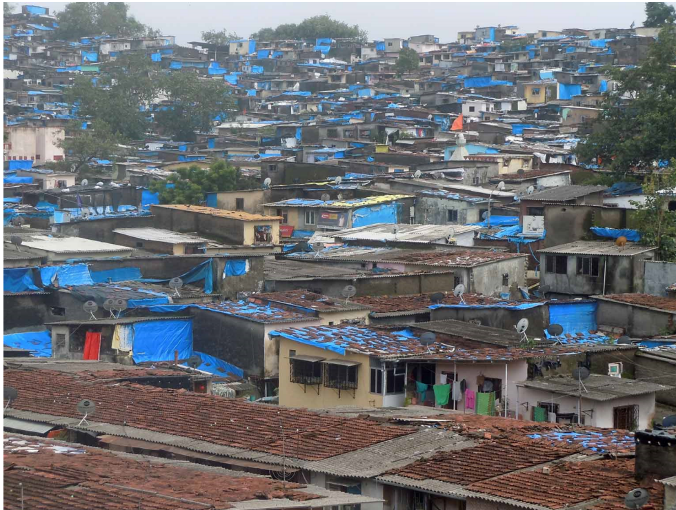
Photo 124. Walls are not always watertight either. The use of tarpaulins is so widespread it turns whole neighborhoods blue. Note the tiled roofs in the foreground, which do not need plastic sheets once they are entirely covered. Asapha, Mumbai, July 20, 2014.
