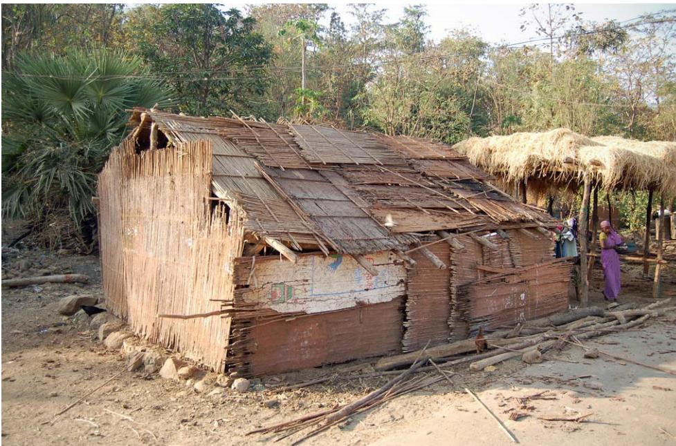
Photo 33. This makeshift house is profoundly kacca as it is made of readily available kacca demolition waste. Kelthan, January 18, 2013.
