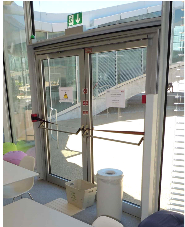
Photo 217. 'Do not use this door!' is an example of a conflict between formality and affordance. July 2012.
