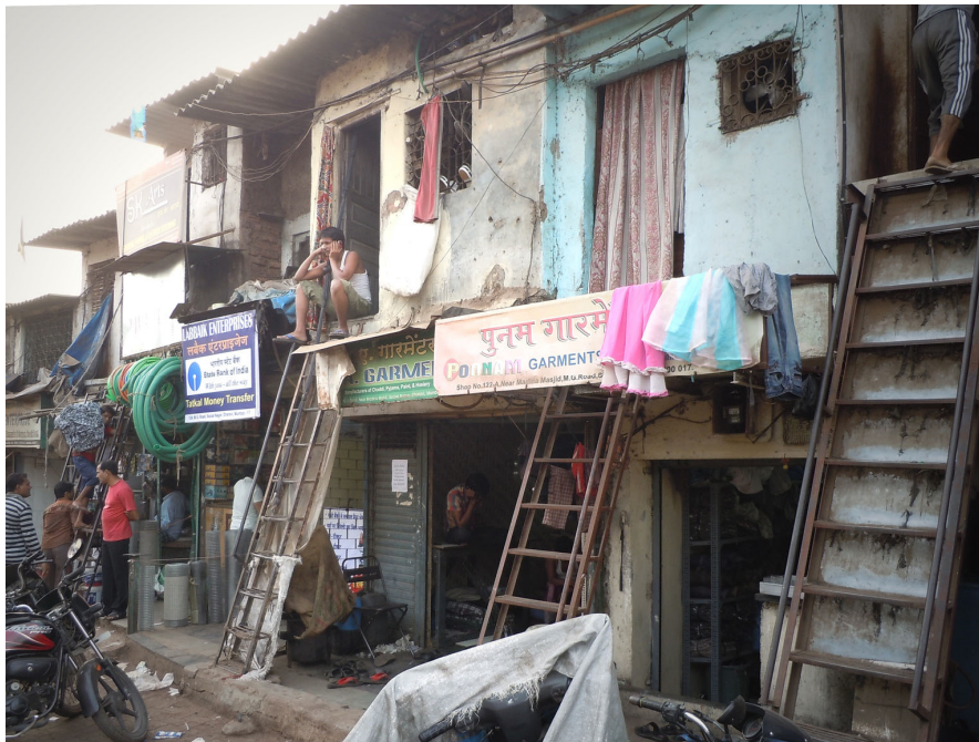
Photo 131. Stairs leading to the first floor front door. January 16, 2013.
