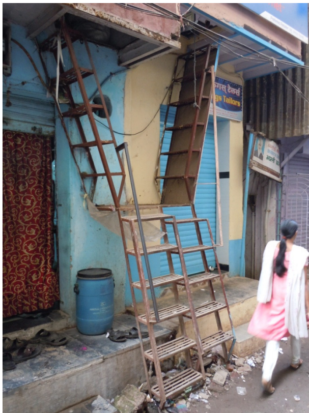
Photo 135. Horizontal neighbors rarely share stairs. The house on the left is older, since both its floor level and the level at which it touches the street, are lower. A white tarpaulin keeps dirt away from the blue water container. January 21, 2013.
