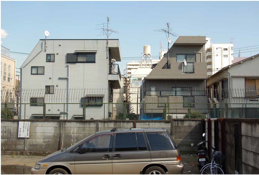
Photo 14. Building volumes restricted by regulations on shadow reduction and height limits. In order to comply, cut offs have been made from the more obvious square shape. The result is un-intentional. Tokyo March 12, 2007.
