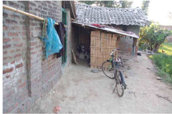
Photo 158. The kitchen is in a kacca annex to the pucca house. August 2, 2014.
