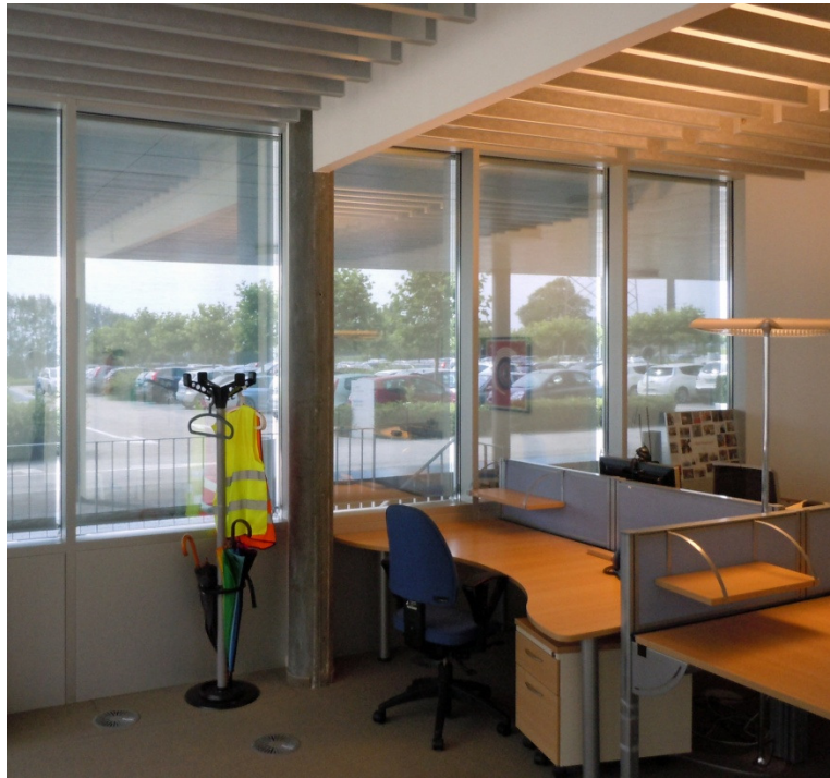
Photo 202. Typical office interior with a raised floor containing ventilation and cabling. July 2012.
