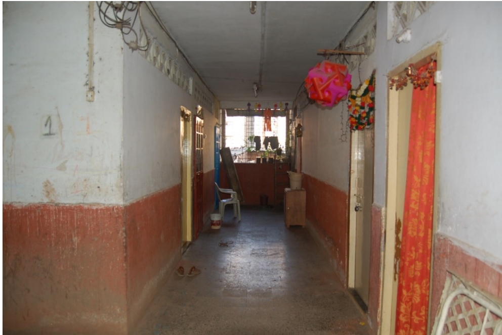
Photo 91. Double loaded corridors do not afford the social life known from living ground-bound in alleys. The space is neither public, nor private, nor common. Dharavi, December 28, 2012.
