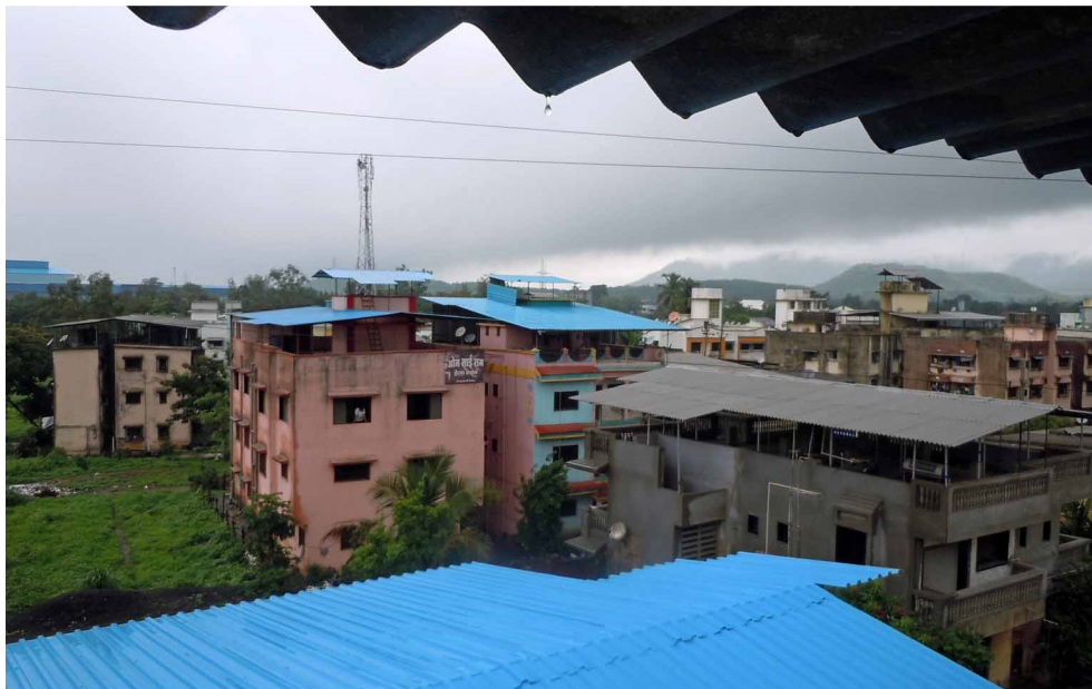
Photo 116. The tin roof over the roof terrace is a modern version of the heat-shield loft. Vasind July 12, 2014.
