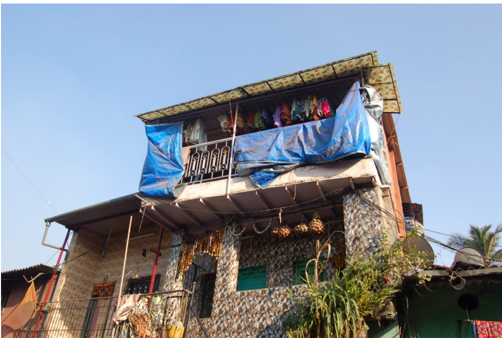
Photo 176. Incremental development also occurs in quality. The façade of this Dharavi mansion is clad with glazed tiles. December 28, 2012.
