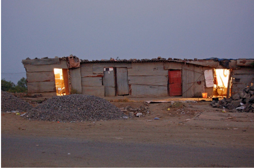
Photo 38. Road workers temporary housing built of corrugated tin sheets. Alibag, January 13, 2010.
