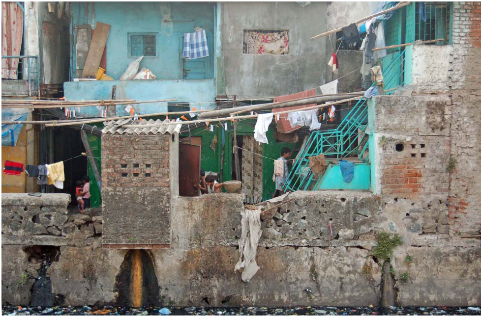
Photo 70. Boys check a detached toilet in Navrang compound. This toilet discharges directly into a branch of Mahim Creek and is therefore independent of sewerage systems or water supply. January 15, 2009.
