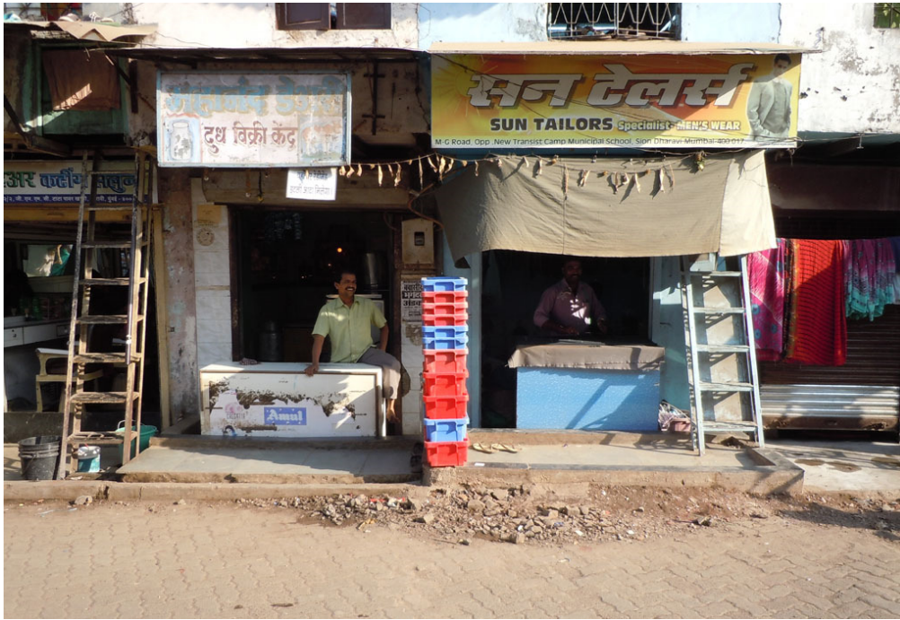
Photo 103. Raised terraces and thresholds will keep the water out during monsoon. The counters 'sink' behind them. The barbershop on the far left uses a one-foot board. January 19, 2013.
