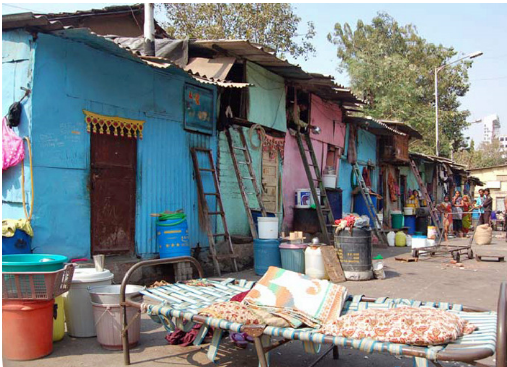
Photo 48. N.M. Joshi Marg, Byculla, Mumbai. Pavement dwellings are becoming more and more pucca . These dwellings are quite permanent as also the neat use of paint is telling. All of them have a loft. January 20, 2010.
