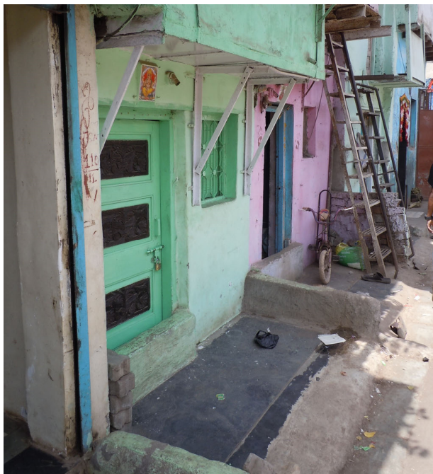
Photo 104. Heightened thresholds keep the water out, but lower the doorway. April 19, 2013.
