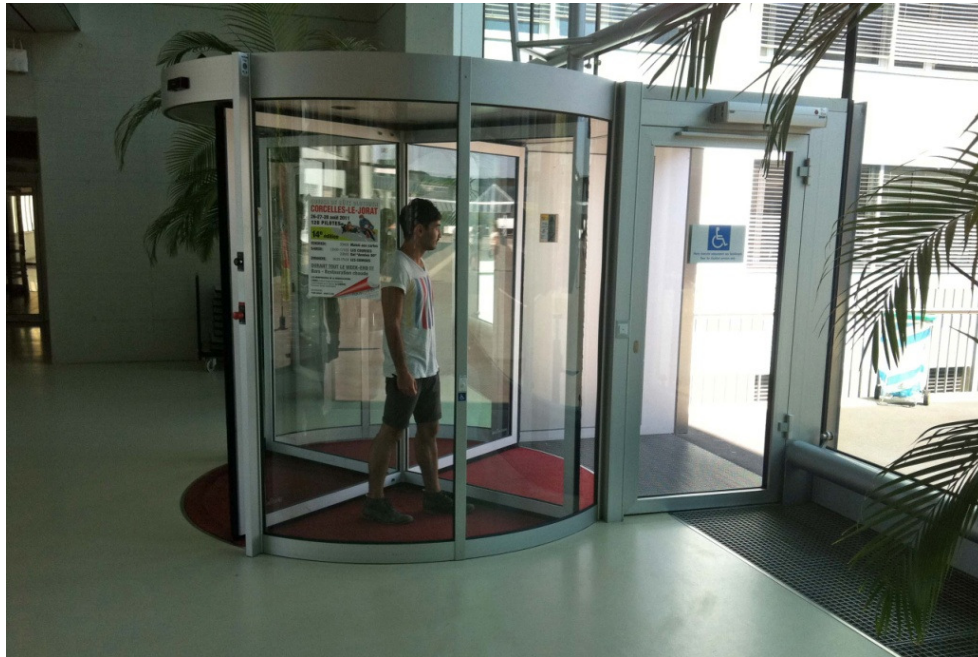
Photo 2. This twenty-first century revolving door autonomously processes a man out of the building. Touching the door will interrupt the process and leave the man stuck in the machine. Note the 'normal' door on the right, for 'disabled people only' as the sign says. September 9, 2011.
