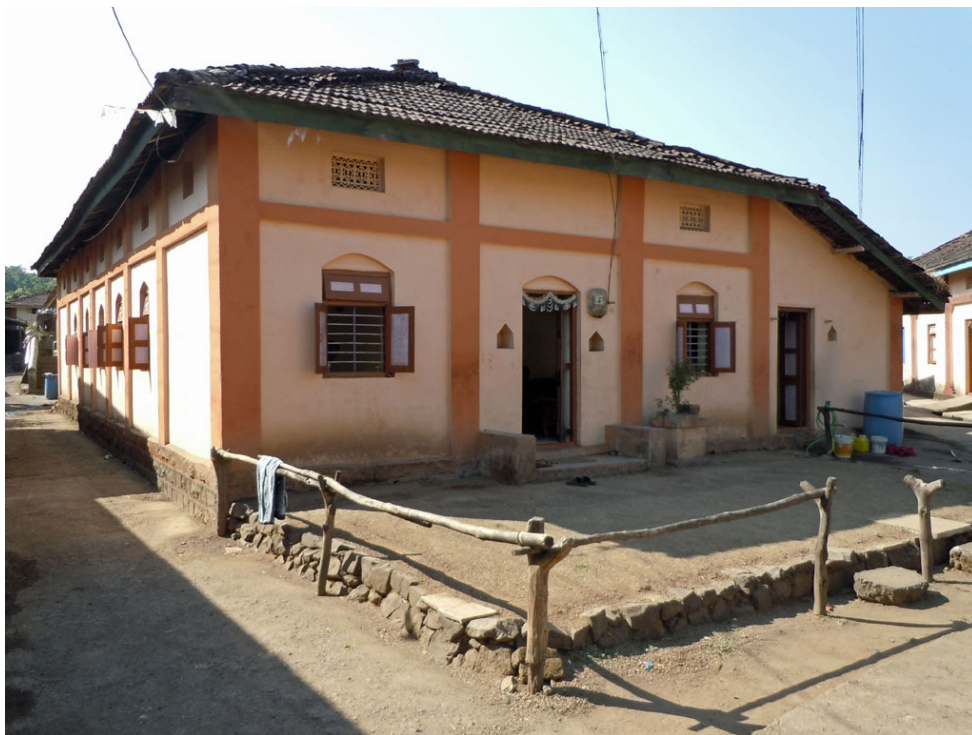
Photo 113. A traditional house in Pundhe, consisting of a ground floor cum loft. The grills under the eaves afford cross ventilation through the loft. November 8, 2012.
