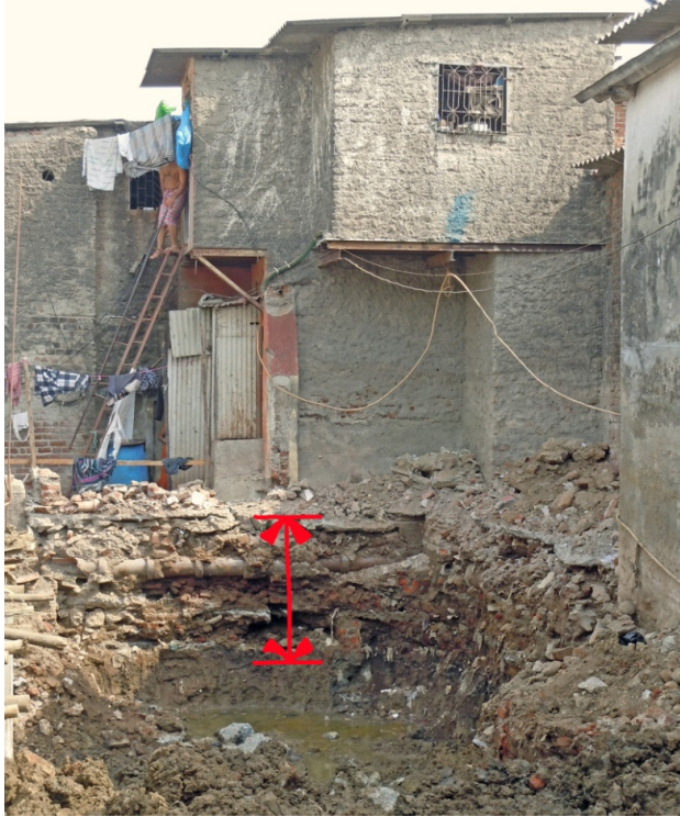
Photo 101. On this site near 90-Foot Road, today's ground level is almost two meters (red arrows) above the natural underground. April 10, 2013.
