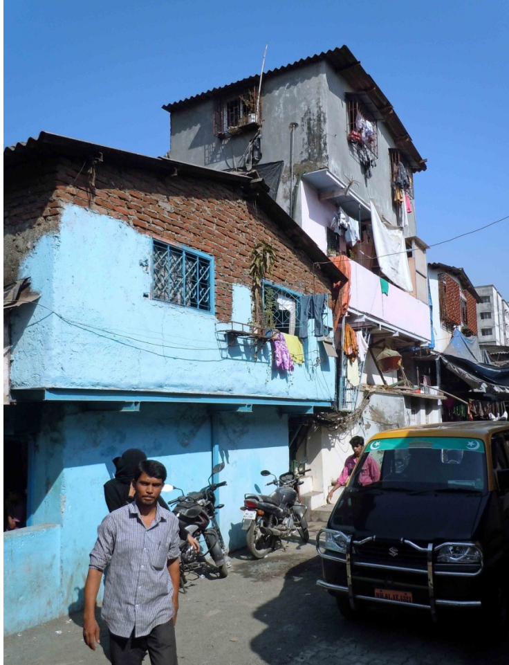
Photo 102. The higher building sits on a higher base and has its first floor level half a story higher than the building on the left. December 21, 2012.
