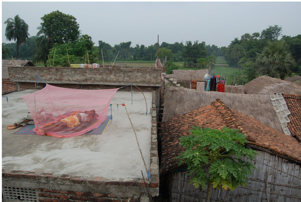
Photo 122. The concrete roof of the pucca house affords comfortable outdoor sleeping, whereas the same concrete slab traps the heat of the day inside. The interior climate of kacca houses (on the right) is generally better. August 2, 2014.
