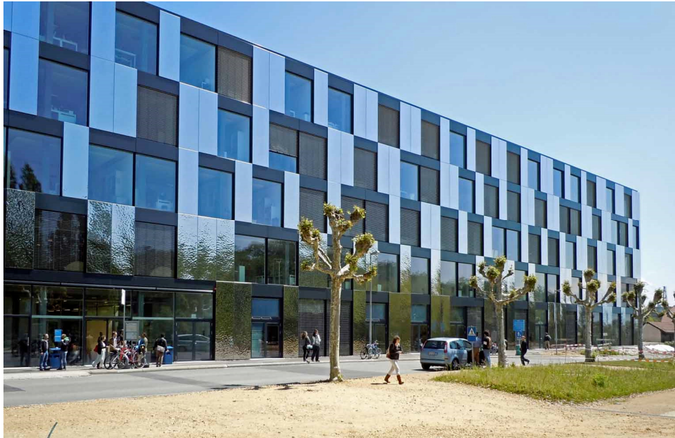
Photo 218. Géopolis, recently built on the Lausanne University campus. September 2, 2013.
