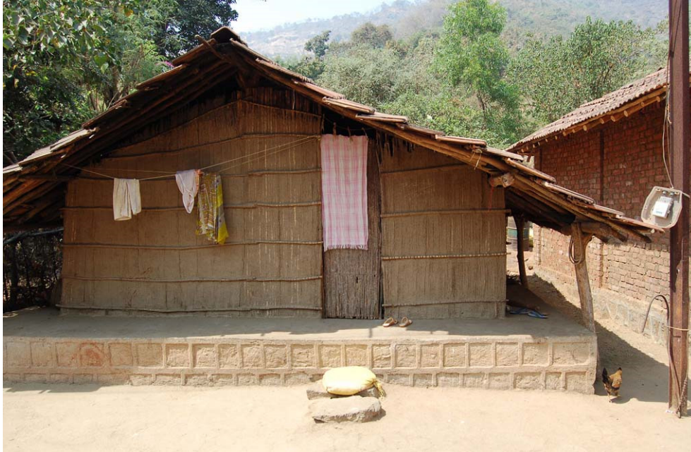
Photo 23. A combination of kacca and pucca . The walls of matting plastered with earth and cow dung are kacca , whereas the roof tiles and cemented base are pucca . Tara, February 21, 2010.
