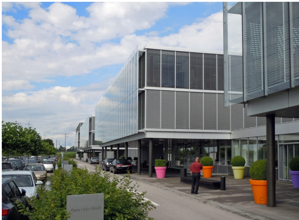
Photo 201. The business center has full glass facades with extra glass screens to the motorway, typical of contemporary architecture. July 2012.
