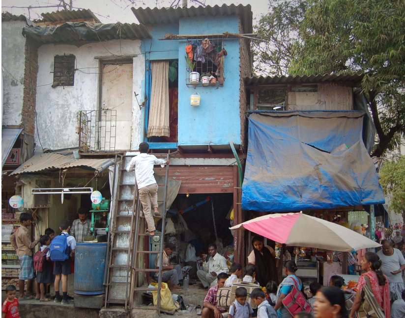
Photo 132. Stepping out of a door onto steep stairs is less comfortable than down through a stairwell. January 20, 2010.
