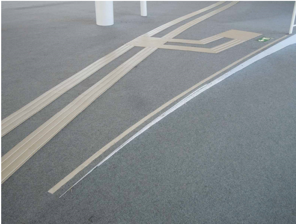
Photo 213. ‘Sensitive’ and fragile details are typical of the RLC. A ramp transforms into a flat floor along an edge ending in infinite thinness. The result is inevitably flimsy, and symptomatic of the disconnection of design from building practice. July 2012.
