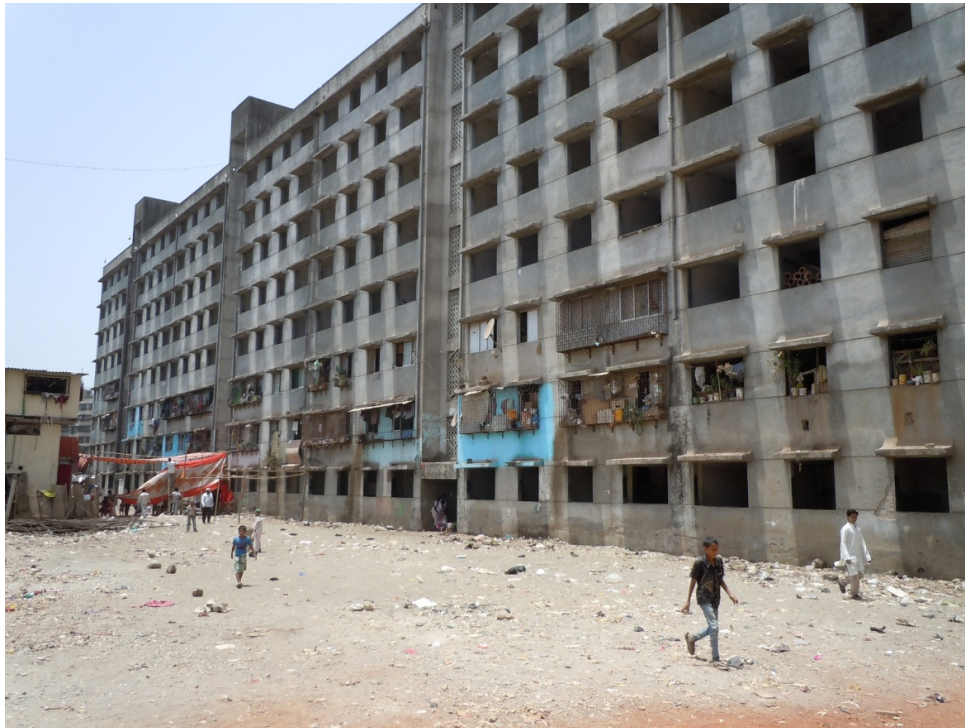
Photo 199. In Kolya Khata building at the heart of Dharavi, squatters have appropriated the first and second floor, whereas all other floors are vacant since 2005. Kuttiwadi, April 19, 2013.
