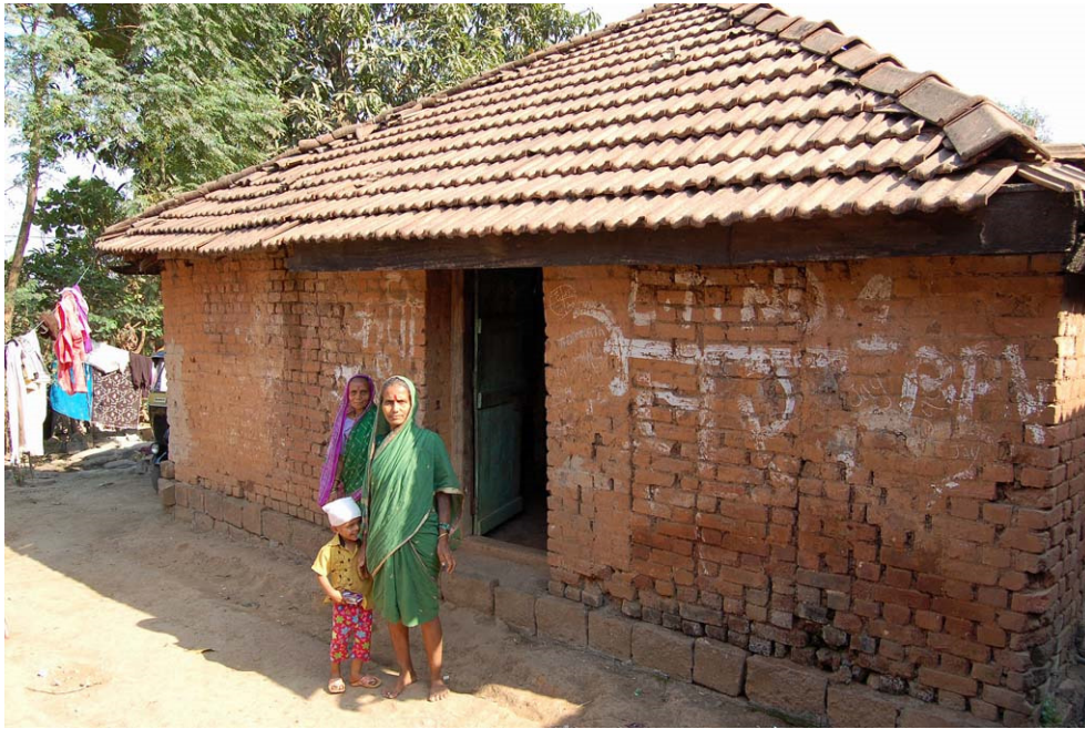
Photo 25. Earth mortar affords easy changing of a facade, as is visible from the traces of the former doorway on the right. Near Vasind, February 27, 2010.
