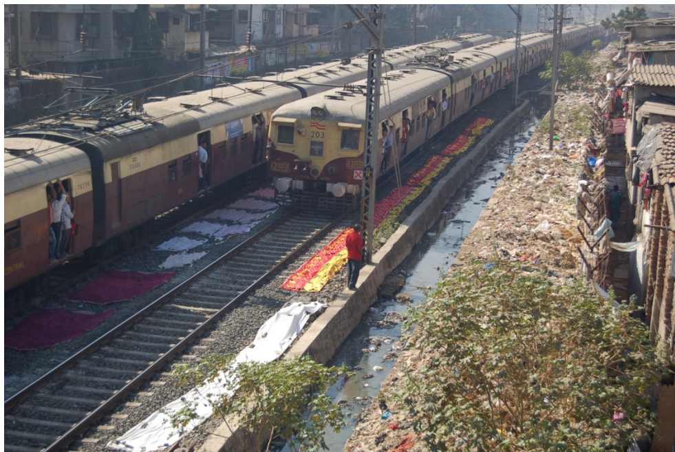
Photo 178. A wall with barbwire separates the slums from the railway land, i.e. a physical boundary marks the formal boundary. Still, launderers use the railway beds for drying, which is an example of kinetic encroachment. January 4, 2013.
