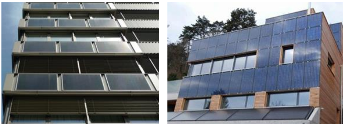
Fig. 5+6: Photovoltaic integration with standard sized panels or custom-made panels.
