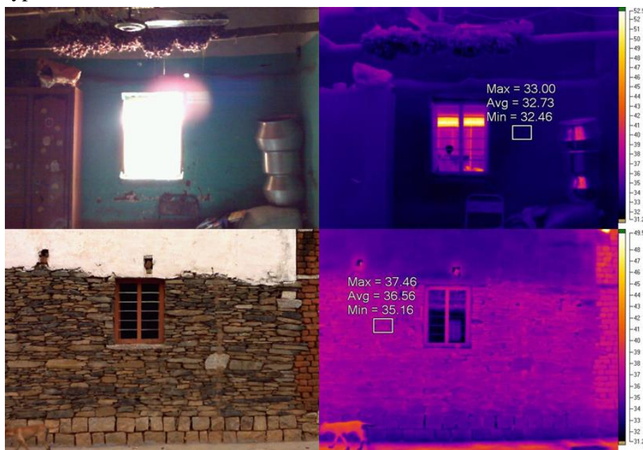
Figure 5: IRT of West wall 1- Indoor surface (top) and outdoor surface (bottom)
