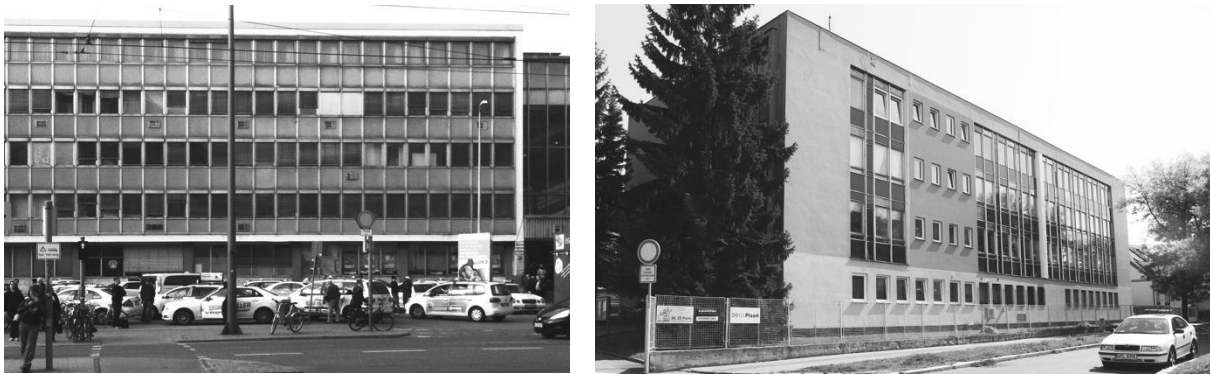
Figure 1: Typical representatives of the target typology – buildings with envelope made of light panels. Left: Main train station in Munich, Germany. Right: Elementary school in Pilsen, Czech Republic. Façade segment with smaller windows already replaced.
