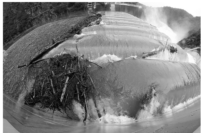
Fig. 1. Malarce Dam (F) PKW during the November 2014 flood event with debris blocking at its right part (photo: EDF France)
