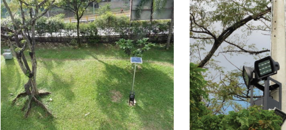
Figure 2: left) Photovoltaic panel installed in the University Campus. right) External ultra-efficient LED illumination point, powered by photovoltaic panel.
