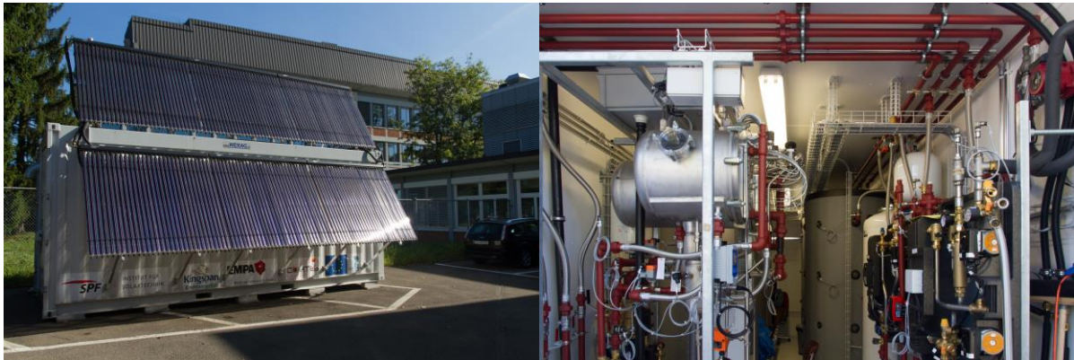
Figure 1: Left: Picture of the complete system from the outside. Solar collectors with an active area of 18\text{ m}^2 are mounted on top and on the side of the shipping container. Right: Picture of the complete system from the inside. On the left is the heat and mass exchanger assembly, with the sorbent and sorbate tanks in the back, and on the right are solar pump station, fresh hot water station and floor heating pump, in the back the sensible hot water tanks are placed.
