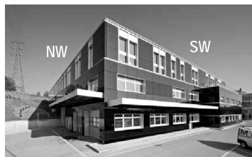
Figure 2: Northwest and southwest facades of the pilot building
