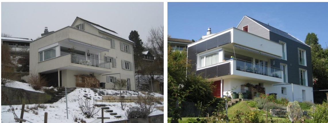
Figure 1: SFH Sulzer before the retrofit (left) and after the retrofit (right).
