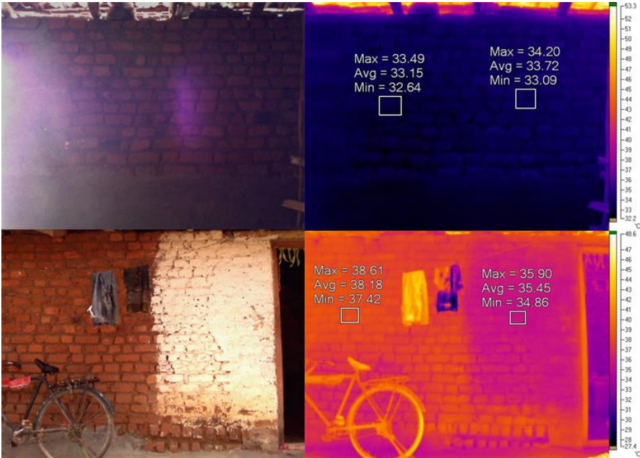
Figure 7: IRT of front wall- Indoor surface (top) and outdoor surface (bottom)
