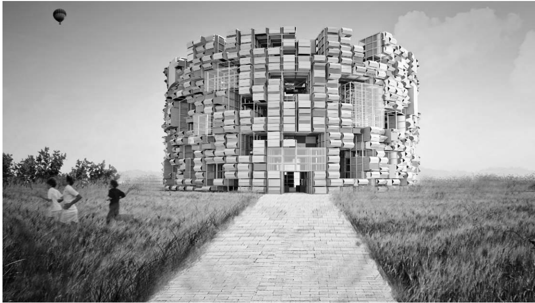
Fig. 2. This project is based on the concept of a modular building, with an external dynamic surface and solar shading devices. The building can grow with the necessity of functionalities. Several functions are included such as a restaurant, a supermarket, a library, a little space for music, flats and offices and commercial destinations are studied in a concept of a vertical city. Credits: D. Pedrini, L. Pilati
