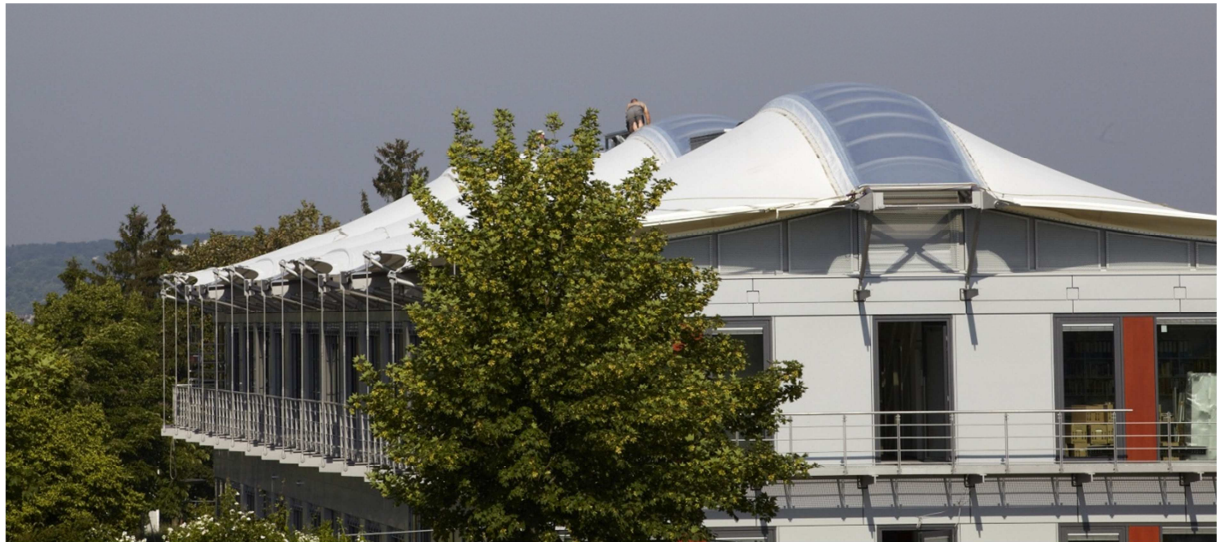
Figure 1: Energy Efficiency Center viewed from south-east. Clearly visible is the textile roof with translucent PTFE-glass membranes and partially transparent ETFE films.
