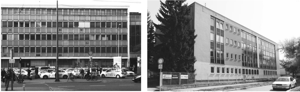
Figure 1: Typical representatives of the target typology – buildings with envelope made of light panels. Left: Main train station in Munich, Germany. Right: Elementary school in Pilsen, Czech Republic. Façade segment with smaller windows already replaced.
