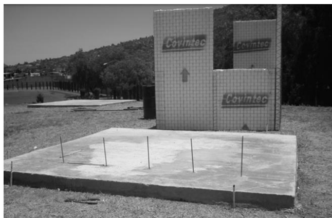
Figure 4. Experimental Modules. Construction process and arrangement
