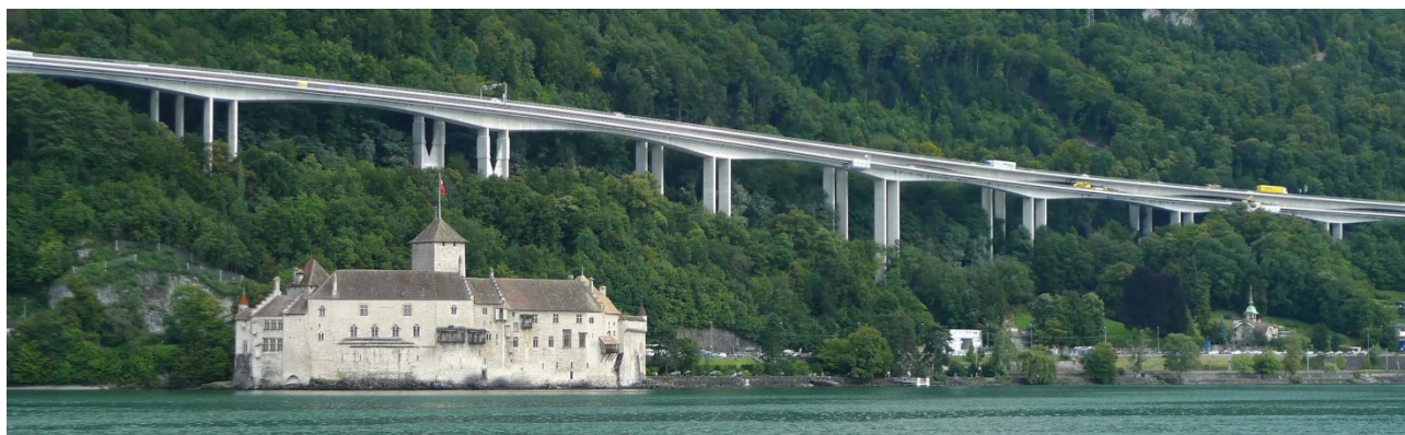
Figure 1 Chillon viaducts along Lake Geneva
