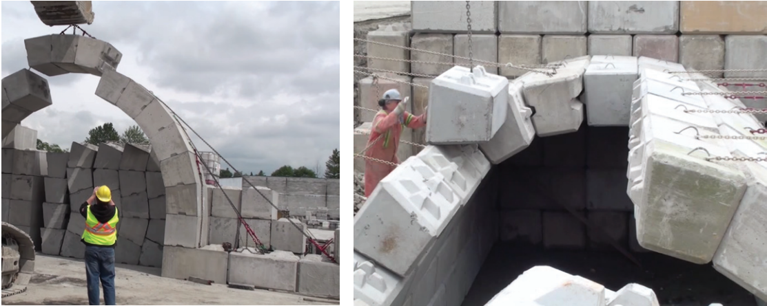
Figure 5.2 – The Arch-Lock system [Dre13] is used to construct a simple arch (left), and a barrel vault (right). [Copyright photographs: Lock-Block Ltd. 2013]
