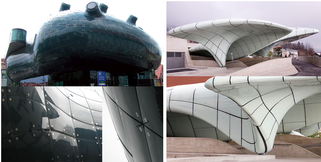
Figure 4.2 – Projects involving double-curved panels where a separate mold has been built for each panel. These examples illustrate the importance of the curve network and the existing difficulties in producing architectural freeform structures. (Left: Peter Cook and Colin Fournier, Kunsthhaus, Graz. Right: Zaha Hadid Architects, Hungerburgbahn, Innsbruck.) Figure taken from [EKS + 10].
