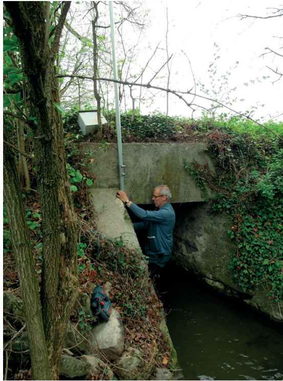
Figure 5.2: Installation of the gaging station Petite Chamberonne .
