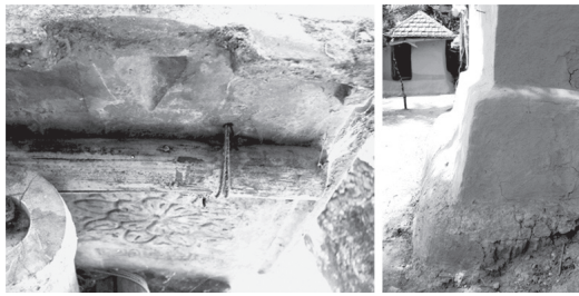
Figure 5. (a) Gayakhali Village (Khulna region): ropes fasten purlins to bamboos arranged above the tiles, creating a continuous connection with the roof structure. Credits: A. Caimi. (b) Hashkhali Village (Khulna region): local floods influence the double step shape of the plinth: the lower step matches the level of the most frequent floods, limiting possible necessary repairs to this small part; the second step is sized in relation to the level of exceptional floods. Credits: A. Caimi.
