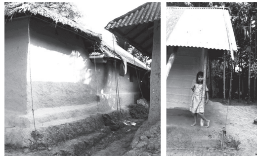
Figure 6. (a) Thakurbad Village (Khulna region): at the four corners of the roof, wall plates are connected by ropes to stakes driven into the ground. Credits: A. Caimi. (b) Ujanbarapait Village (Sylhet region): gable roof anchoring system with bamboo arranged above the CGI sheet covering and connected to stakes driven into the ground. Credits: A. Caimi.
