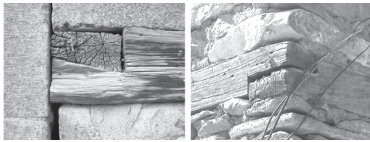
Figure 2. (a) Special halved corner joint with double dovetail in Erzurum City (Republic of Turkey). Credits: M. Hofmann. (b) Ordinary halved corner joint in Cumahkızık Village (Republic of Turkey). Credits: M. Hofmann.
