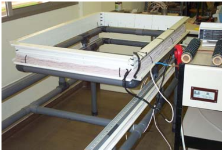
(a) Transformer realised in the university of Saragosse [68]
