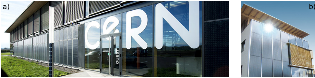
Figure 1.2: (a) Solar façade at the "centre d'entretien des routes nationales" (CERN) in Bursins, Switzerland. Credits: ENERGIE SOLAIRE SA. (b) Façade installation with glazed solar thermal collectors. Credits: WINKLER SOLAR GMBH
