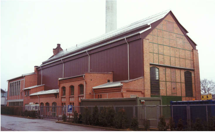
Figure 2.1: Example for a building retrofit with a reddish coloured solar thermal installation in Göttingen, Germany. Credits: SOLARWALL ®
