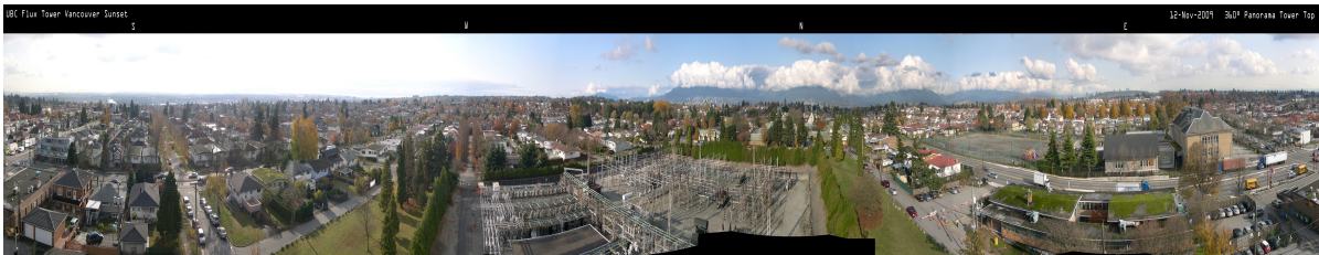
Figure 3.1: Panorama picture of the neighbourhood ‘Sunset’, taken from the top of the Urban Climate Research Tower. Image kindly provided by Prof. Andreas Christen. Photographer: Rick Ketler, Geography Dept. at UBC.
