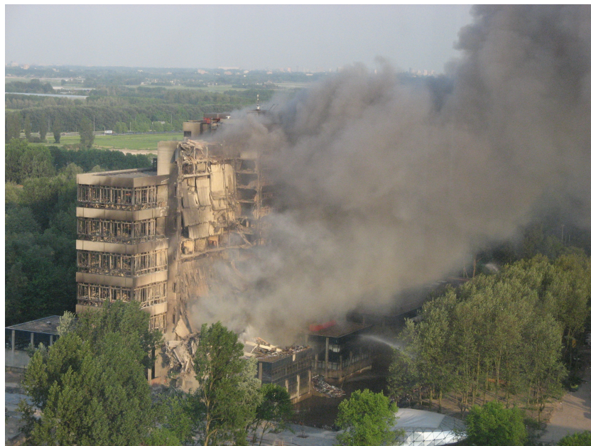
Figure 2 – As a consequence of a short circuit, a building of the architecture faculty in Delft burned down [Minh, 2008].
