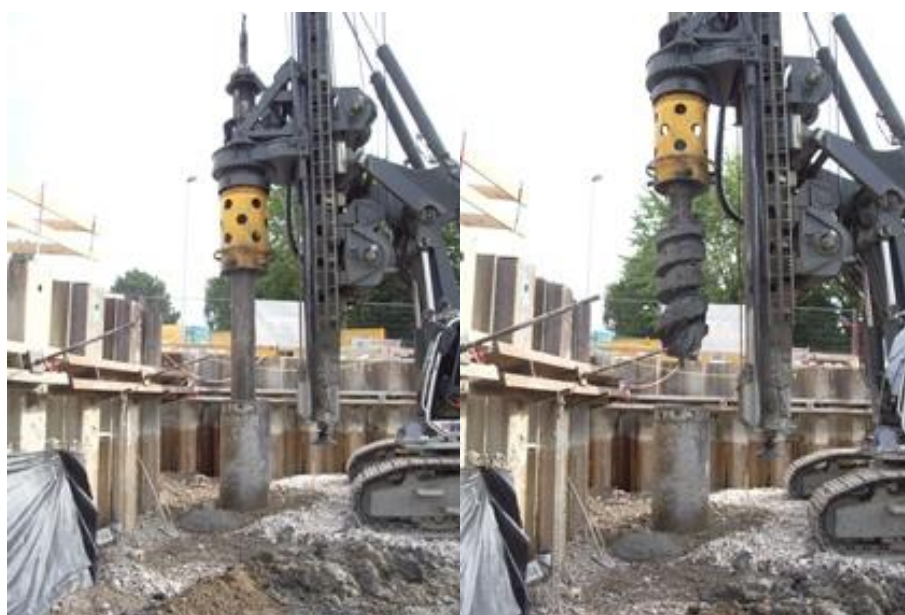
Figure 9:20 Augering of pile #3
