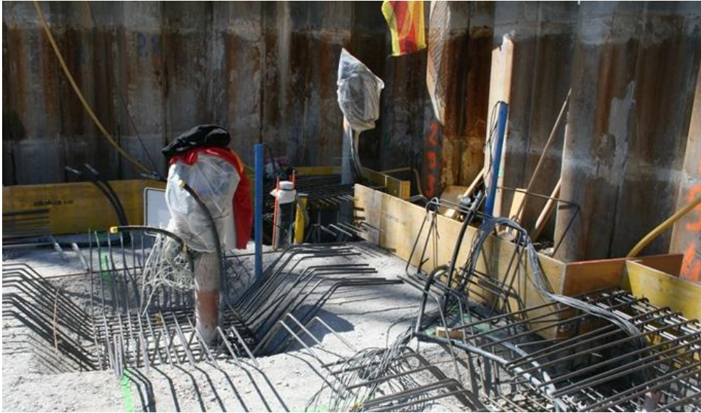
Figure 9:25 Installation of the reinforcing rods in the raft
