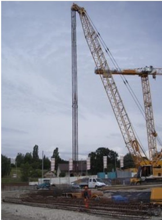
Figure 9:21 Lifting of an equipped 28 m long reinforcing cage
