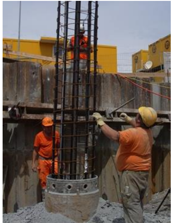
Figure 9:22 Insertion of the reinforcing cage into the temporary casing
