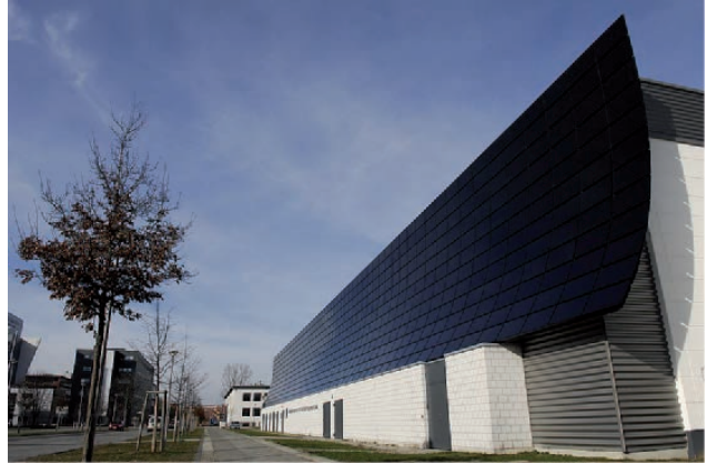
Fig. 15: Ferdinand-Braun-Institute, Berlin: 732 dark CIS modules designed as a curved façade (Surface: 640 m 2 , Energy output 39 kWp, System Provider: Sulfurcell Solartechnik GmbH, 2007)
