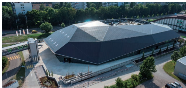
Fig. 1: Umweltarena Spreitenbach (Switzerland 2012): an example of a 203% PlusEnergy building achieved by means of a customized 750 kWp full-roof BIPV skin consisting of c-Si panels with an anti-reflective glass (Architect: René Schmid Architekten; System provider: 3-S Photovoltaics, Meyer & Burger Group; Photo: Bruno Helbling)
