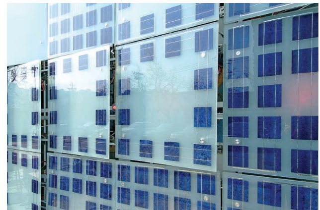
Fig. 45: Media Wall at Xicui entertainment complex, Beijing (China): combining sustainable and digital media technology, featuring the world's largest colour LED (2008)
