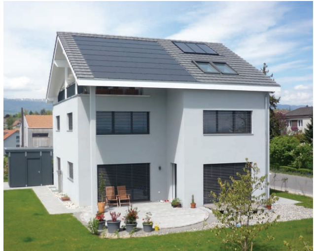
Fig. 20a: Frameless c-Si in-roof installation, Ins (Switzerland): 32 modules (Surface: 35 m 2 , Energy output: 5.12 kWp, System provider: 3-S Photovoltaics, Meyer & Burger Group, 2011; Courtesy: Derk Bätzner, Photo: P. Heinsteint)
