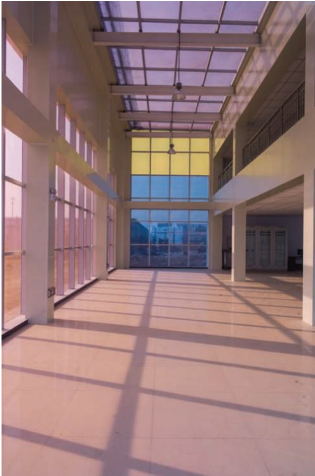
Fig. 43: Boading (China 2012) semi-transparent a-Si modules with coloured polymers (Courtesy: Tianwei Solar Films; Photo: P. Heinstein)
