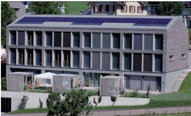
Fig. 23: In-roof installation combined with cement fibre panels (Courtesy: 3-S Photovoltaics, Swisspearl)
