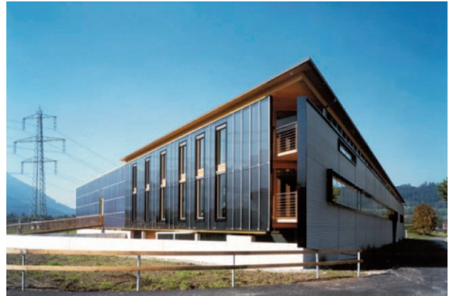
Fig 4: Energiepark West, Sattels (Austria): Early and well-designed example of a 150 m 2 c-Si solar façade (Architects: heim + müller architektur zt gmbh; Photo: Christine Kees, 1996)
