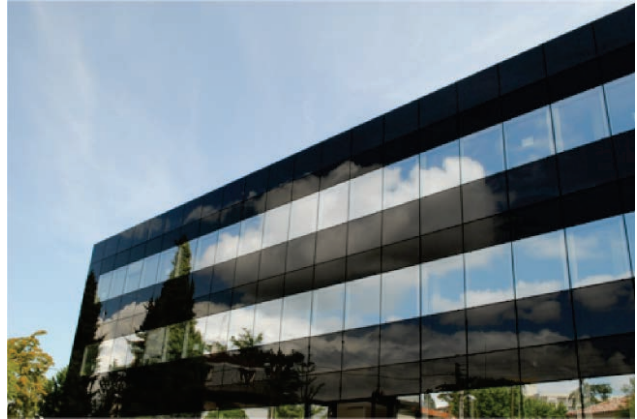
Fig. 34: Rhône-Alpes area (France): PV façade with micromorph thin-film PV panels of 1.10 \times 1,30 \text{ m} each (ou bien: 1.4 \text{ m}^2 ) (Surface: 130 \text{ m}^2 ; Energy output: 738 kWh; System provider: Pramac; Façade: Face InTec, 2011)
