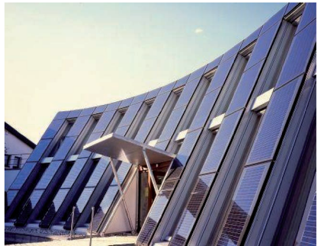
Fig. 30: Juwi Head Office, Bolanden (Germany): ideal façade inclination with large-scale PV modules to harvest a maximum of solar energy (Surface: 70 m 2 , Energy output: 7.2 kWp, System provider: Schüco International KG, 2004)
