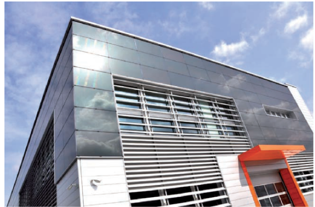
Fig. 9: Albasolar Head Office, Alba (Italy): the exterior of the building consists of an amorphous photovoltaic ventilated façade (System provider: Albasolar, 2012)
