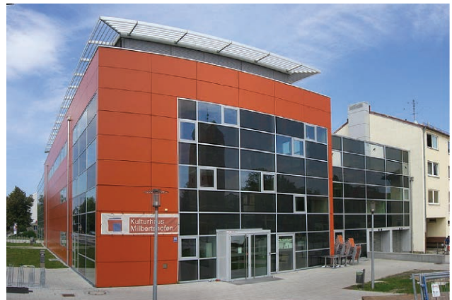
Fig. 31: Kulturhaus Milbertshofen (Germany): façade with black micromorph and semi-transparent thin-film modules (Energy output: 3 kWp), RPM-Architekten, System provider: Voltarlux, 2008)
