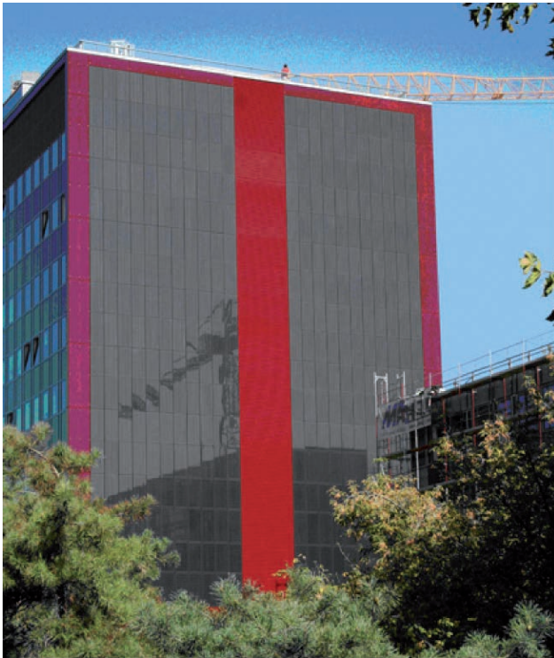
Fig. 29: Building of the Chamber of Commerce, Vienna (Austria): mono-c-Si façade (Surface: 447 m 2 , Energy output of 55 kWp, (Architect: Eduard Neversal Ziviltechniker GmbH; System provider: Ertex-Solar, 2008)
