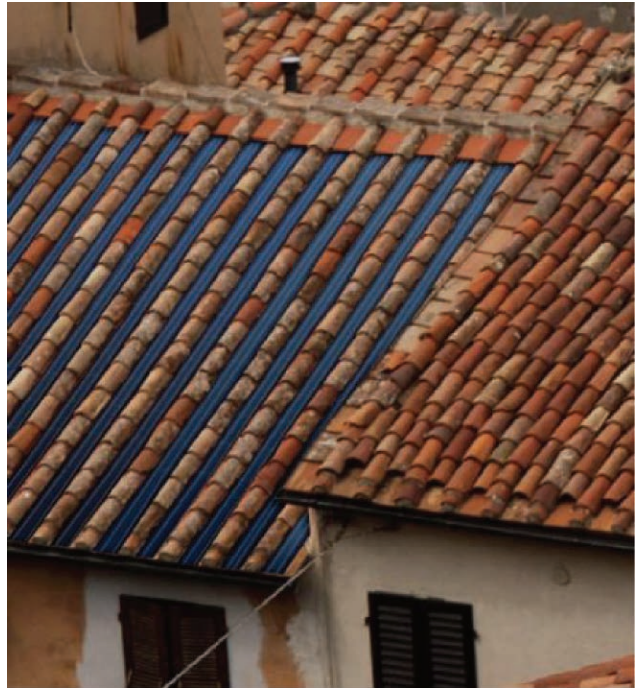
Fig. 28a: Solution by vertical installation of PV panels on Mediterranean roofs (System provider: Hemera)
