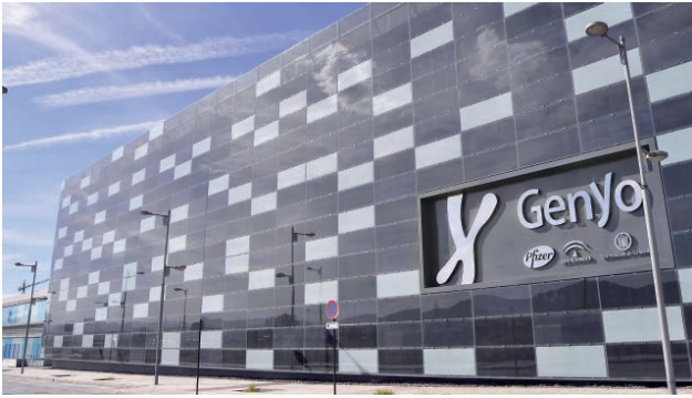
Fig. 36: Pfizer-University of Granada-Junta de Andalucía Center for Genomics and Oncological Research (Spain): the ventilated solar façade combines PV elements (2,5 × 1 m each) with serigraphic glass, both specially customized for this project (System provider: Onyx Solar, 2010)
