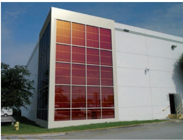
Fig. 17: Façade with dye sensitized cell (DSC) technology (System provider: Konarka, 2011)
