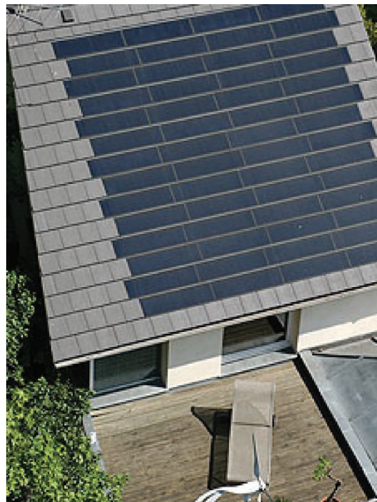
Fig. 25: Solar shingles: ideal for shale roofs (System provider: Solar Century)
