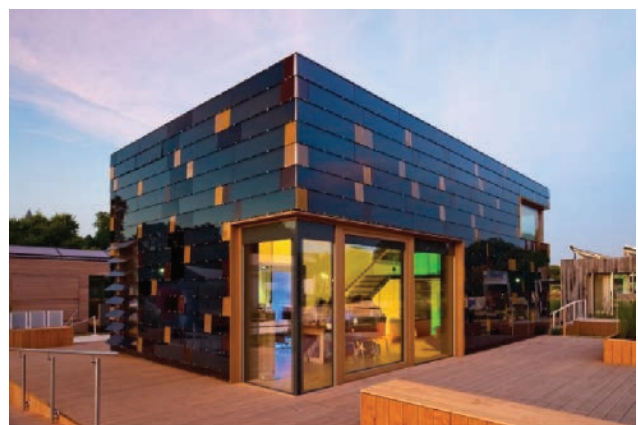
Fig. 32: Solarhaus Darmstadt (Germany): prize-winning pilot project from the Technische Universität Darmstadt with a 200% PlusEnergy gain. The façade is covered with black CIS thin-film modules (System provider: Würth-Solar, 2009)
