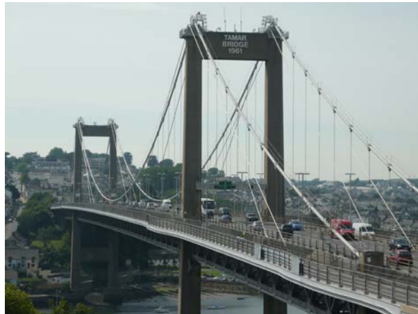
Figure 3. The Tamar Suspension Bridge
