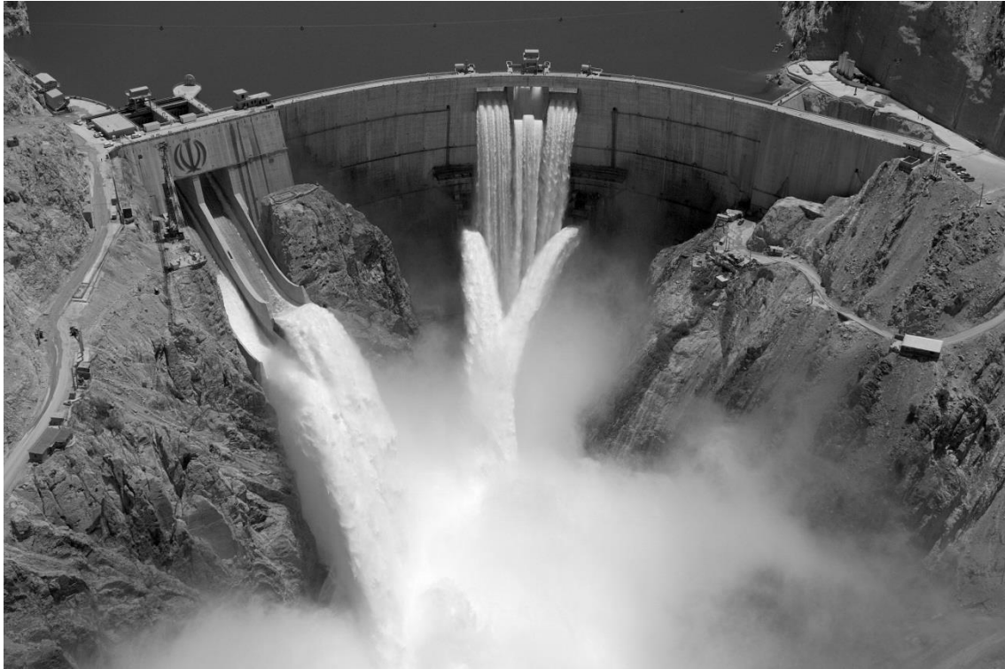
Figure 1.1. Spillage at Karun III dam in Iran, example of simultaneous use of different jet trajectories and tailpond dam (Photo Iran Water & Power Resources Development Co., 2010).
