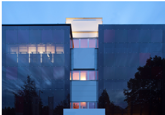
Figure 1.4: Example of a photovoltaic wall, by the German company MASDAR PV.
