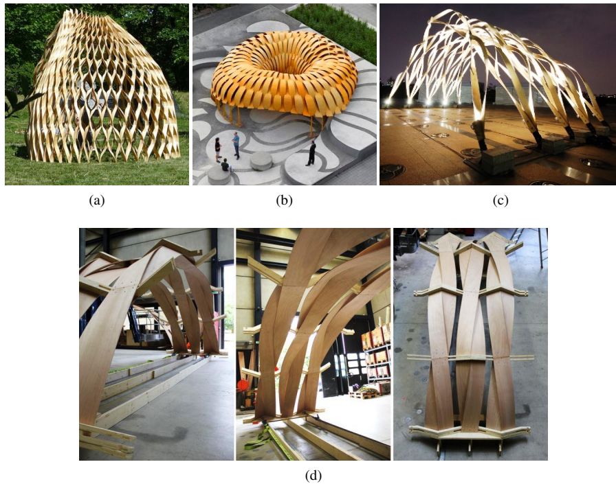
Figure 3: Interlaced form-active structures made from flexible panels: (a) The wood Pavilion of Oslo School of Architecture and Design, (b) ICD/ITKE research pavilion 2010, (c) The "Radical Wood Pavilion" (d) Timber Fabric Structures: photo © Markus Hudert
