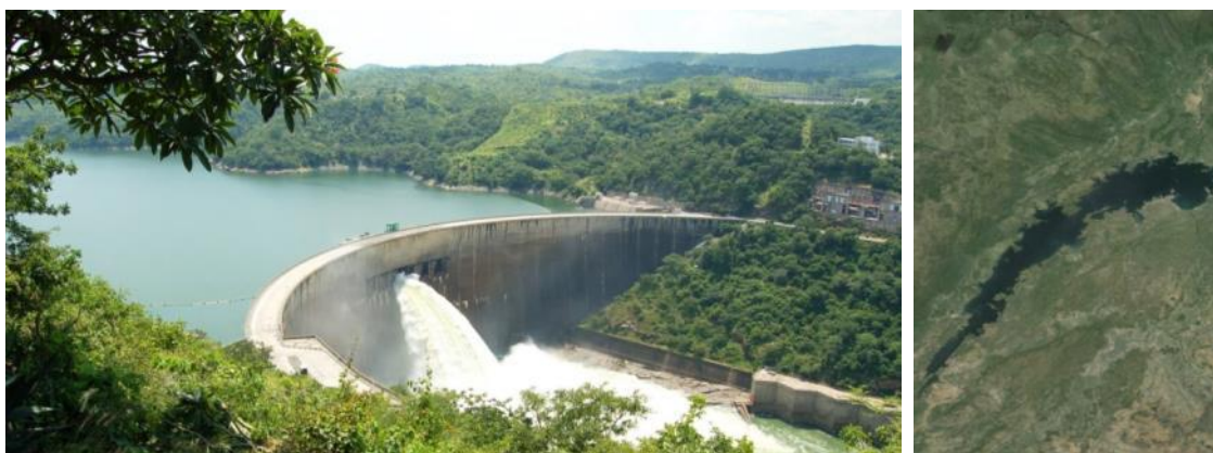
Figure 2.7. Kariba dam and reservoir (left photo by Sean Ross, from Panoramio: http://www.panoramio.com/photo/65334783 ; right image from Google Earth – approx. 210 km across).
