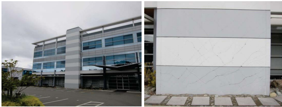
Figure 5 Observed distress to a concrete wall with minimal damage (Photos: Courtesy of Elwood)
