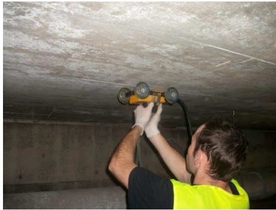
Figure 7. Locating rebars using a GPR system.
