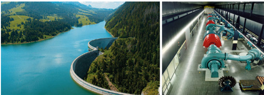
Fig. 1 Hongrin reservoir with the twin-arch dam (left) and view of the existing 170 m long Veytaux 1 powerhouse (source www.alpiq.ch )
