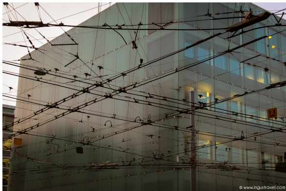
Figure : BNP Paribas Building in Geneva 1
