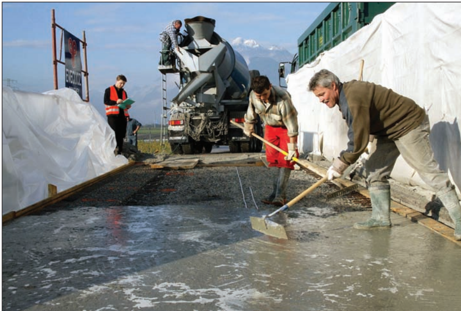
Fig. 8: UHPFRC casting and handling of UHPFRC using simple tools
