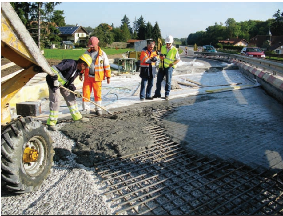
Fig. 15: UHPFRC casting for R-UHPFRC strengthened zone over a pier
