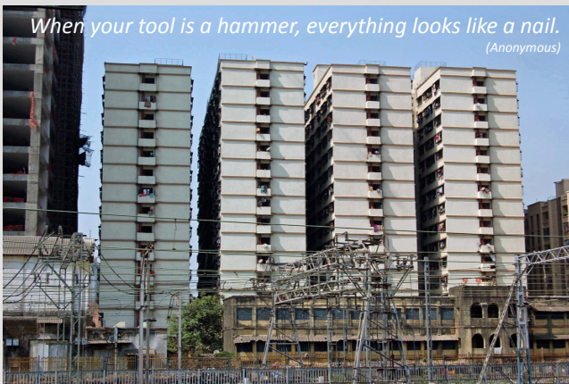
When your tool is industrial production, even housing looks industrially producible. Inhabitant-excluding development.
