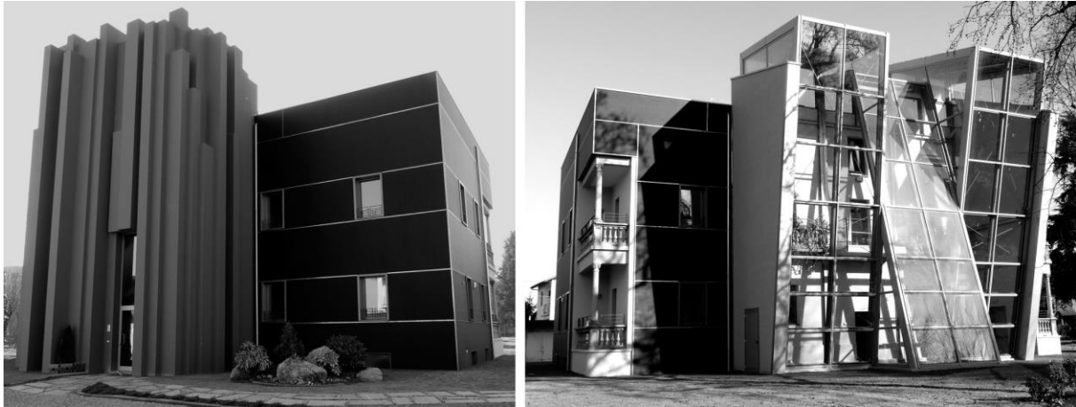
Figure 2: North view (left) and South view of the building after the intervention (right).
