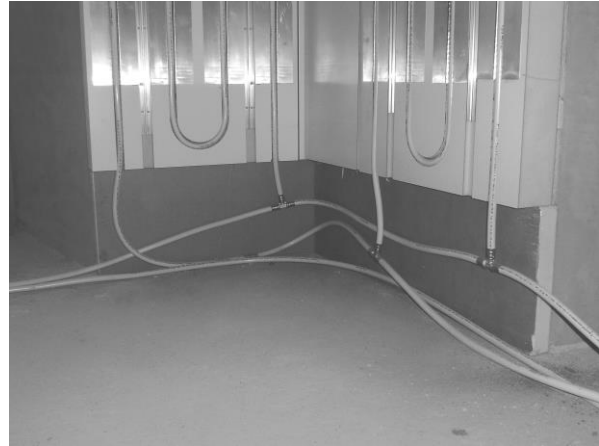
Figure 2: Hydraulic connections of the pipes
