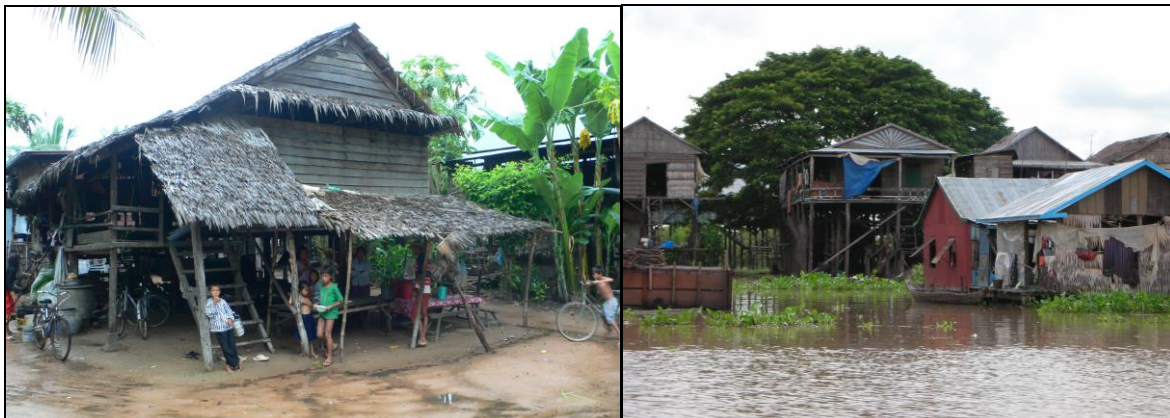
Figures 1a and 1b : Traditional rural Khmer houses with wooden poles. The building serves as a shelter. During the day the house functions as a large umbrella. Work and life go on at ground level, where the most effective shade is provided. At night, people sleep upstairs
