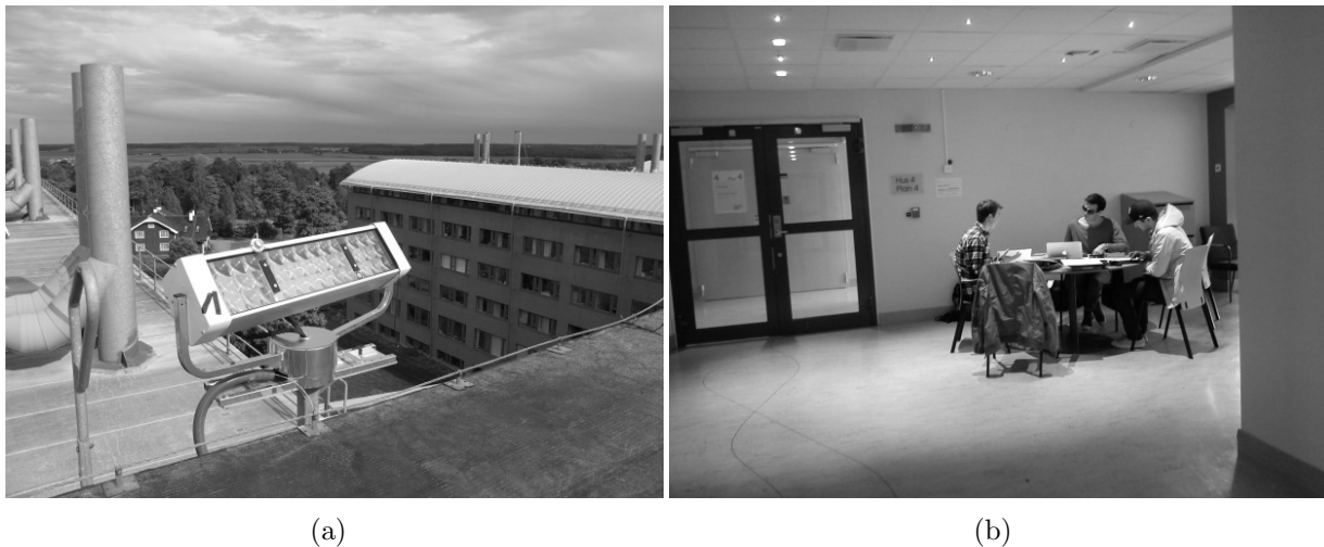
Figure 1: (a) The sun-tracking solar light collector of the SP3 system. (b) The study hall area, where the solar fiber optic light luminaires of the Parans SP3 system have been installed, shown during a sunny day in May 2012. The electric lights have been dimmed down.
