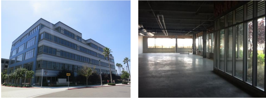
Figure 2: Unoccupied office building for measurement. (Left) Exterior appearance; (Right) Interior space
