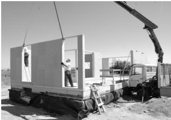
Figure 7: view of the house in construction Figure 8: structure of wood and sheep's wool
