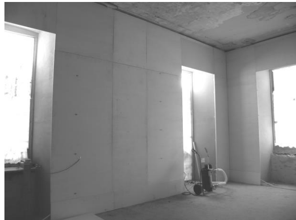
Figure 4: Thermal performance monitoring phase of the pilot room
