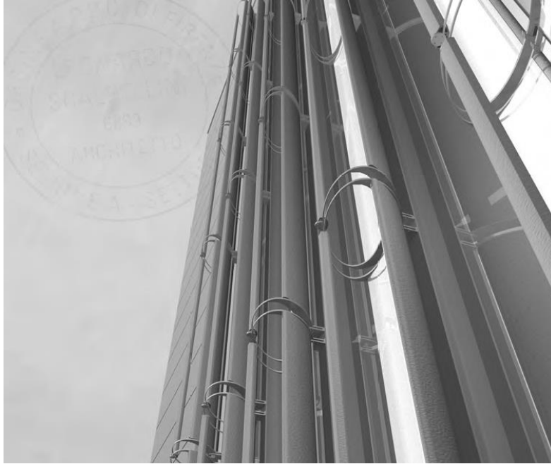
Fig. 5 -View of architectural integration in south facades. Different solution for vertical and horizontal PV concentrator - shading systems are provided.
