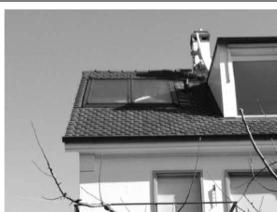
Figure 2: Test system on an inclined roof. Source: Lützelschwab GmbH
