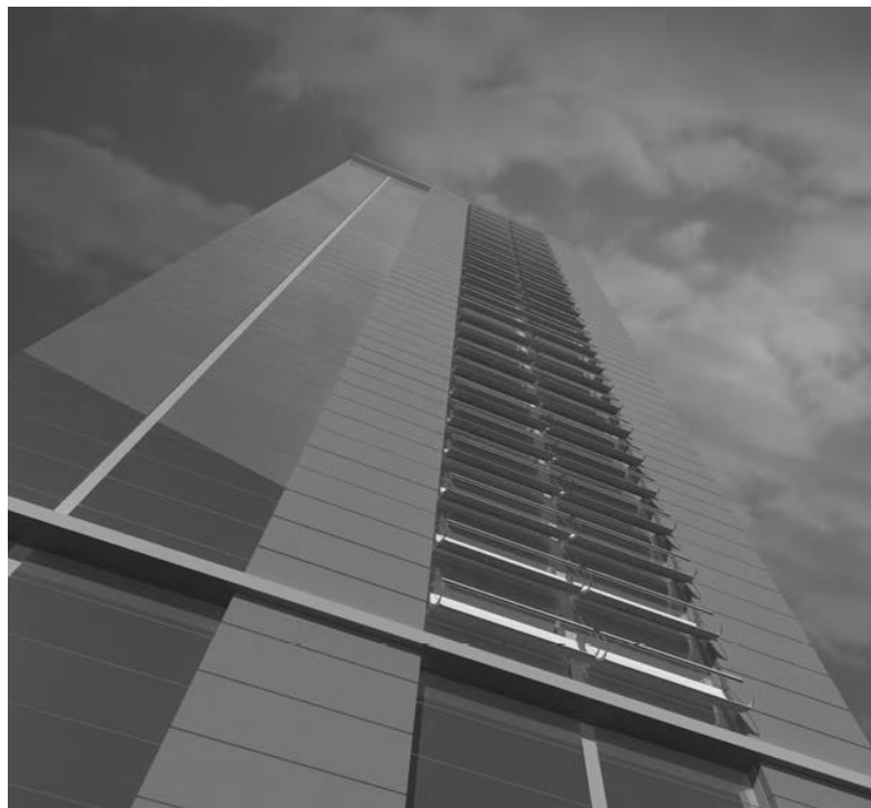
Fig. 6 View of architectural integration in east-west facades.
