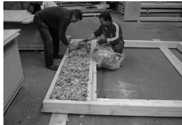
Figure 7: view of the house in construction Figure 8: structure of wood and sheep's wool
