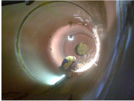
Figure 9 Welding of the diaphragm inside the connection tunnel
