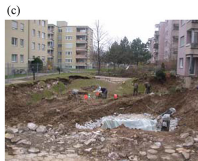
Fig. 1—Structural collapses due to punching shear failures in Switzerland: (a) shopping center, Serfontana, 1970s (photo courtesy of M. Ladner); (b) underground parking garage, Bluche, 1981 (photo courtesy of R. Suter); and (c) underground parking garage, Gretzenbach, 2004 (photo courtesy of A. Muttoni).
