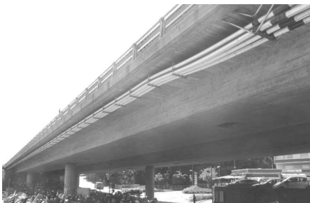
Fig. 1: Morges Highway Bridge
