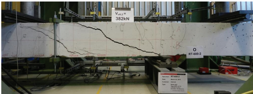
Fig. 4 Specimen RT 600-2 at second failure; first crack was braced after full opening
