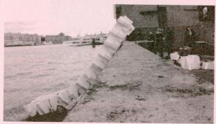
as a flexible post-tensioned polystyrene structure, fastened along the embankment handrail as a hinge, it was reacting to the tidal amplitudes in the Thames River.
