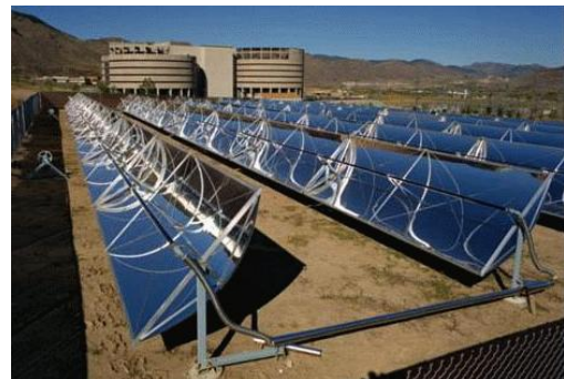
(b) Parabolic trough concentrator array. Source: NREL
