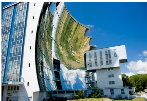
(a) Experimental 1 MW solar furnace at Promes Odeillo, France. ©by David Blaikie
