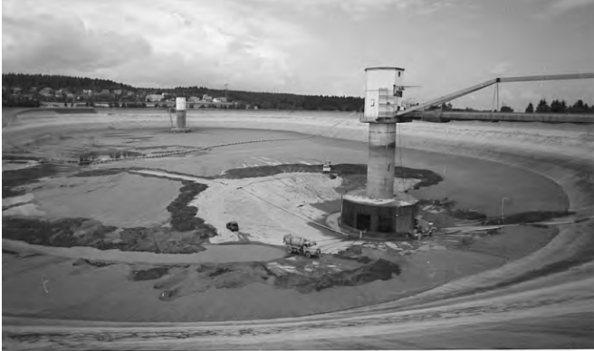
Figure 2.3 Drawdown of Eggberg Basin for sediment removal in 1992 (photo courtesy of G. Klebsattel)
