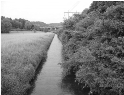
Site B2: Totally channelized, river bed is stabilized with concrete sills in regular distance (System Turnherr)
