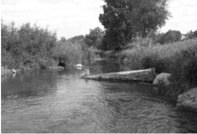
Site B1: Restored site with removal of left bank, insertion of instream structures such as logs and large boulders
