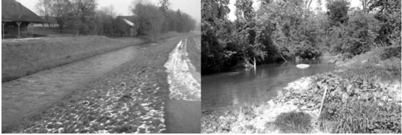
Site V3: Trapezoidal artificial channel with minor structures at river bed (left). Site V4: meandering channel through an alluvial forest (right)
