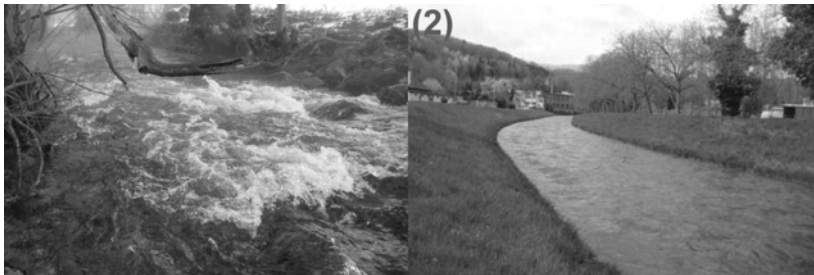
Site V1: straight natural channel with step-pool resp. riffle-pool sequences (left). Site V2: Trapezoidal artificial channel with uniform flow conditions (right)
