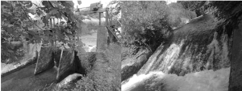
Left: Impoundment for run-of-river plant at Tieffurtmühle (downstream of site n°1). Right: Interruption of longitudinal connectivity due to steep bed stabilizing ramp
