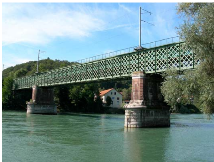
Figure 1. Railway bridge over the Rhine between Koblenz (Switzerland) and Waldshut (Germany).
