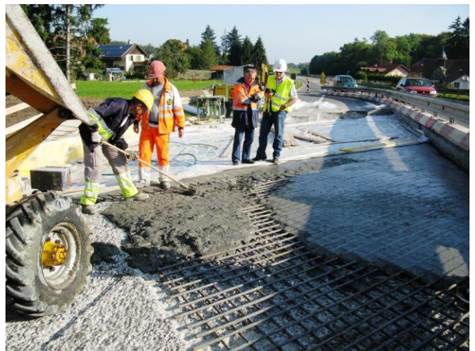
Figure 14. UHPFRC casting for R-UHPFRC strengthened zone over a pier.
