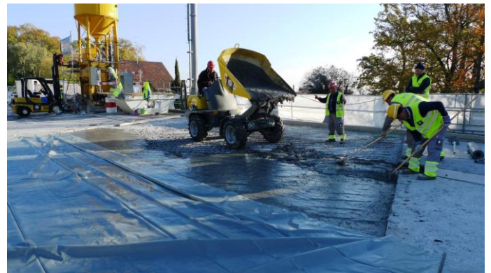
Figure 10. On-site production and casting of UHPFRC.
