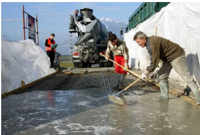
Figure 9. UHPFRC casting and handling of UHPFRC using simple tools.
