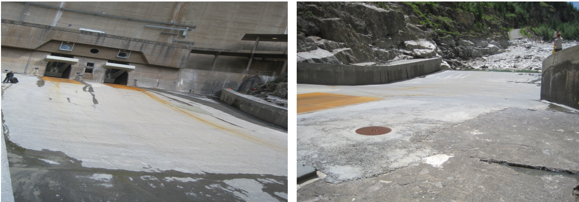
(a) At the bottom of the dam
