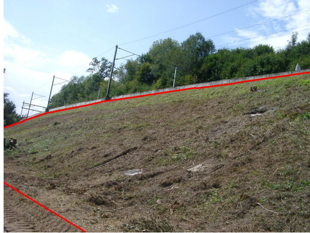
Figure 5.12: Monitored slope at Flamatt
