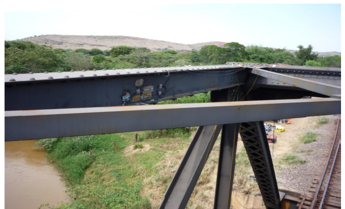
Figure 13. Strain gauges on top chord of truss.
