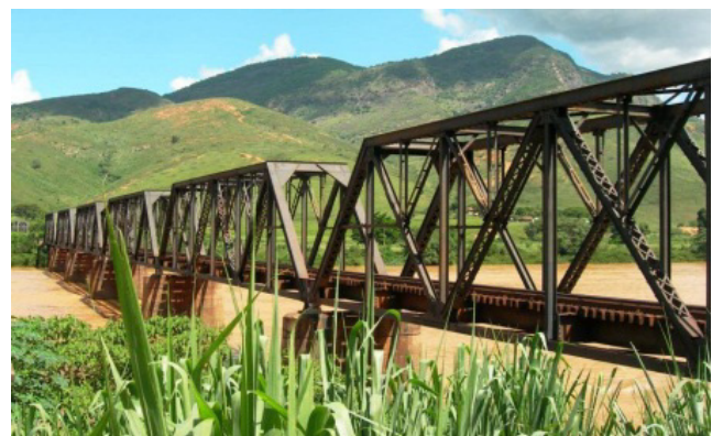
Figure 1. Viaduct composed of single span standard steel trusses.
