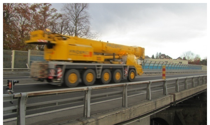
Figure 7. Test vehicle crossing bridge during monitoring system calibration.
