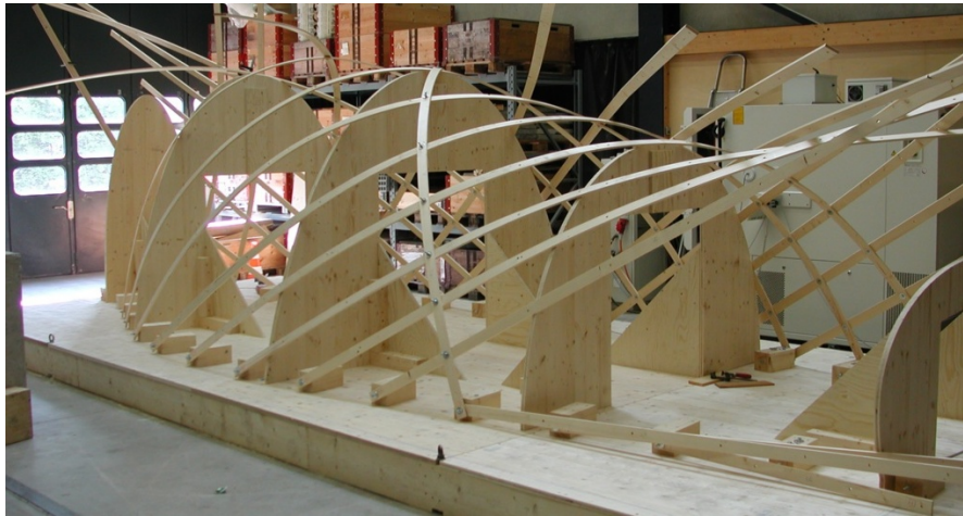
Figure 3.3: Assembling screw-laminated beams for a timber rib shell prototype based on two families of geodesics supported by a third family of vertical planar elements [Pirazzi and Weinand 2006]. Image courtesy IBOIS (EPFL, Lausanne).
