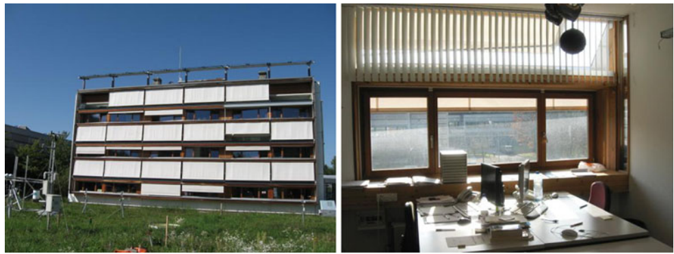
Fig. 1 View of the south façade of the LESO building ( left ) and typical cellular office ( right )
